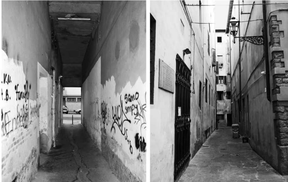
Figure 1.6 – Left. Pistoia. An interstitial space between two buildings used as an underpass (and, when the need arises, as a urinal). Right. Florence. An alley in the historical centre. [Photo: Leonardo Zaffi]
