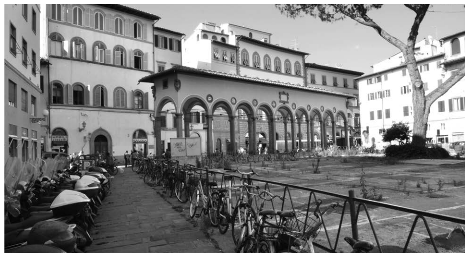
Figure 2.32 – Florence, Piazza dei Ciompi. The square when it was occupied by the Flea Market huts ( above ) and after their demolition ( below ).
