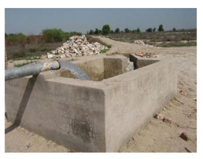
**Plate 3.4** Vertical drainage through installing tube well (an example from Pakistan); the poor quality groundwater is used to irrigate salt tolerant plants at the Biosaline Research Station of NIAB, Pakka Anna near Faisalabad. Gypsum stones are also seen which are used as amendment for mitigating the high SAR and RSC (Residual sodium carbonates) levels of the water
