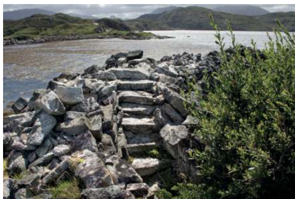
Figure 10.8 View of the stair gallery at Kylesku broch, Assynt (photo: G. Cavers)
