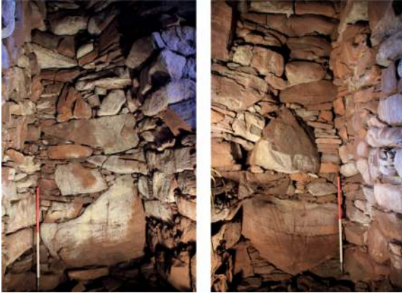
Figure 2B.19 Cell 2 interior, showing the vertical slabbing and horizontal coursing in the south (left) and north (right) walls, which is not integrated with the internal wall of the broch.
