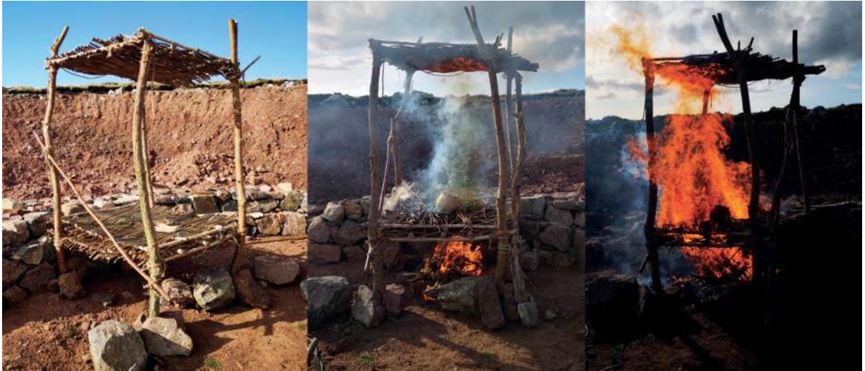
Figure 10.6 The 'test of concept' burning of replica wattle screens against a 1:1 scale model of the broch's inner wall and scarcement, carried out in a quarry at Stoer. The structure burned to destruction in a matter of minutes
