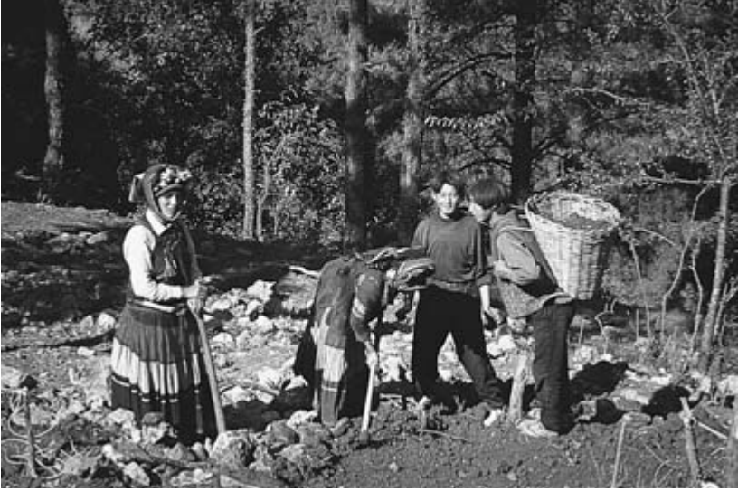
FIG. 13. Nuosu women's clothing as everyday gear: building a road near Guabie
