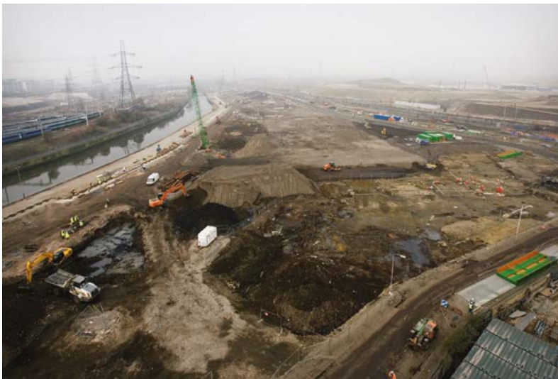
Figure 6.7 Preparing the Olympic site, March 2008. Source: GLA.
