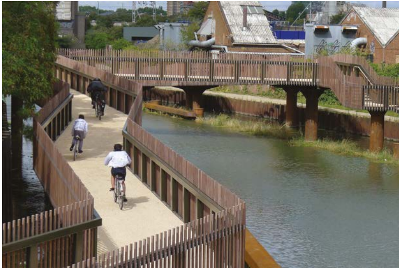
Figure 6.17a Improving connections: floating towpath at Bromley-by-Bow. Source: DfL/GLA.
