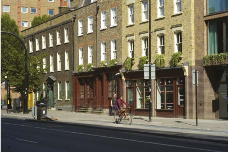
Figure 3.14 High Street 2012: refurbished terrace on Whitechapel Road, illustrating heritage as a key design anchor. Source: Peter Bishop.
