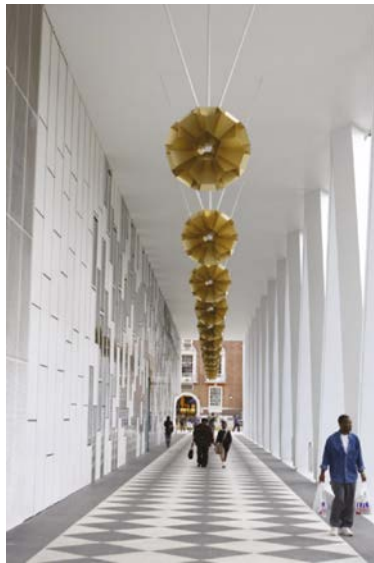
Figure 3.6 Barking town centre arcade beneath affordable housing by AHMM. Source: muf/DfL/GLA.
