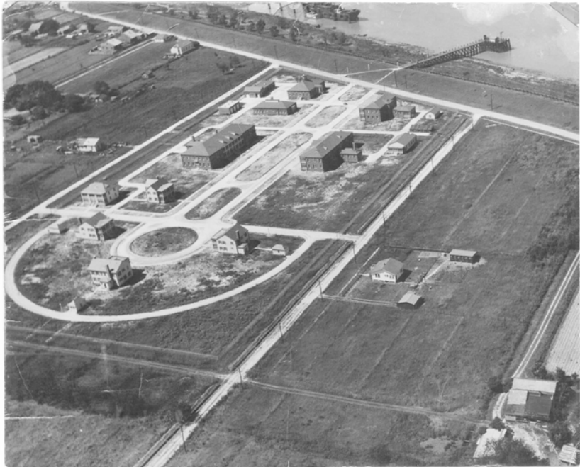
Figure 1: US quarantine station, New Orleans, c. 1930, showing the site's location on the West Bank of the Mississippi River
