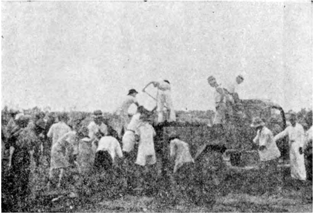
Construction of Airfields (Cooperation from the Local People)
