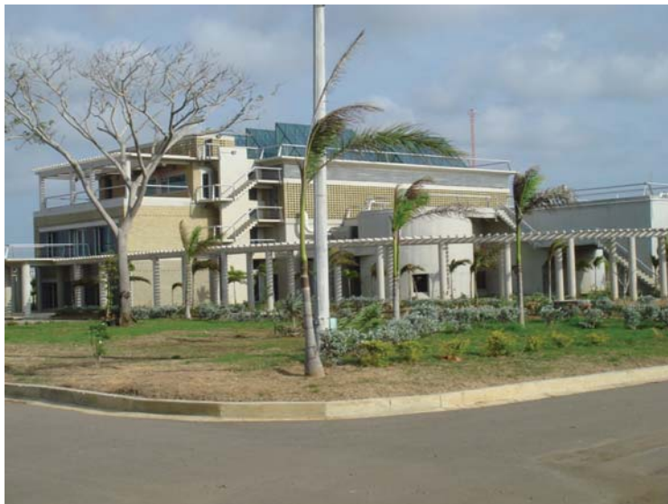
Figure 4.16 The wastewater treatment plant of the city of Cartagena, Colombia, consisting of rotating micro screens and vortex grit chamber, located inside a modern architecture building
