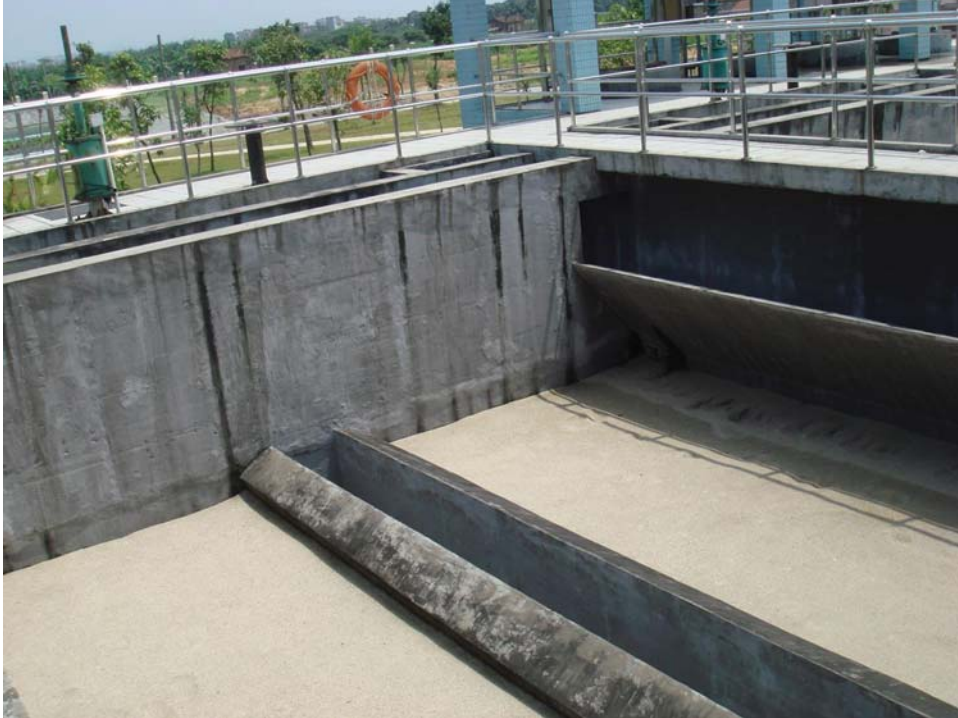
Figure 1.39 A sand filtration unit used for polishing an effluent of an activated sludge plant in the province of Guangdong in China
