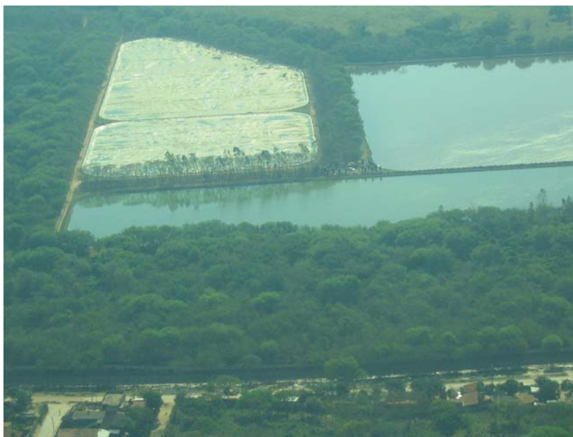
Figure 1.54 The covered anaerobic lagoons in the upgraded N2 lagoons plant in Santa Cruz, Bolivia
