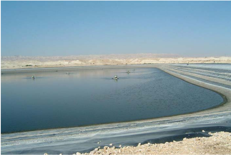
Figure 1.33 Mixers installed in the Og stabilization reservoir
