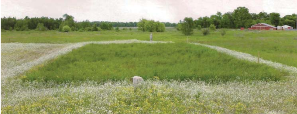
Figure 8.8 Insulated subsurface flow constructed wetland near Oak Grove, Minnesota ( Source: Wallace, 2007)
