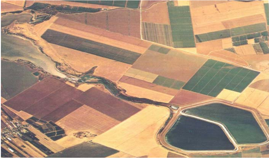
Figure 1.29 Photo of a two cells in series reservoir (Maale Hakishon reservoir)
