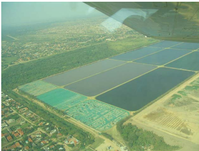
Figure 1.13 Air photo of Plant E after covering the anaerobic lagoons
