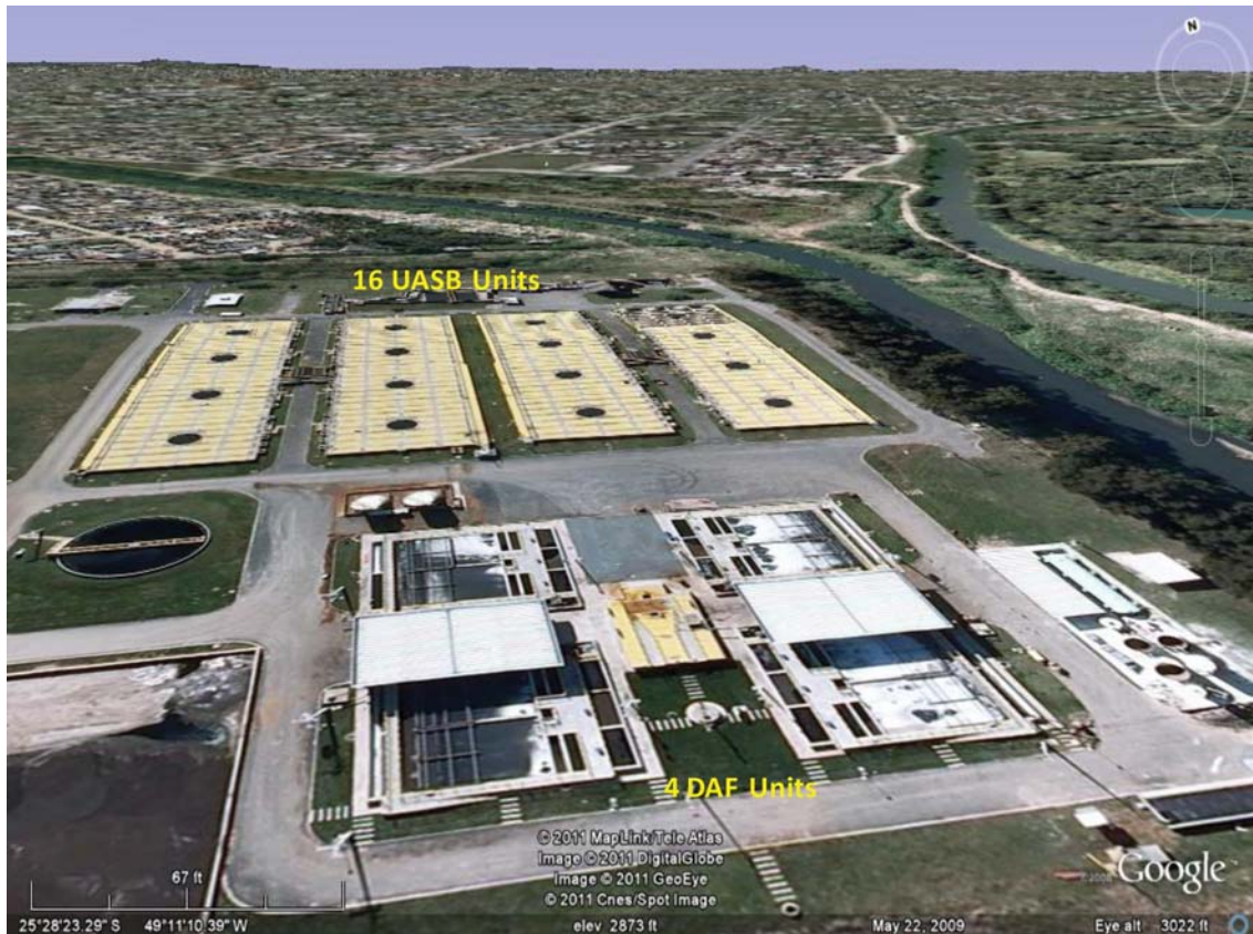
Figure 1.70 The treatment plant Atuba Sul in Curitiba, State of Parana, Brazil, based on UASB followed by dissolved air flotation
