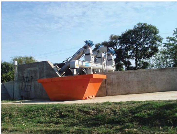
Figure 1.56 The rotating micro screens (RMS) unit serving plants N2 and N1
