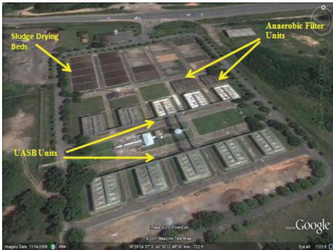
Figure 1.68 The treatment plant of Ipatinga, State of Minas Gerais, Brazil, based on UASB reactors followed by anaerobic filters
