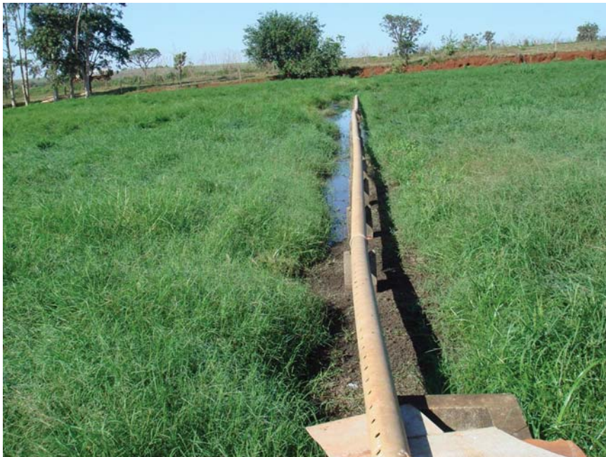
Figure 1.43 One of the wastewater distribution pipelines of the capin overland flow plant in the city of Uberaba, Brazil
