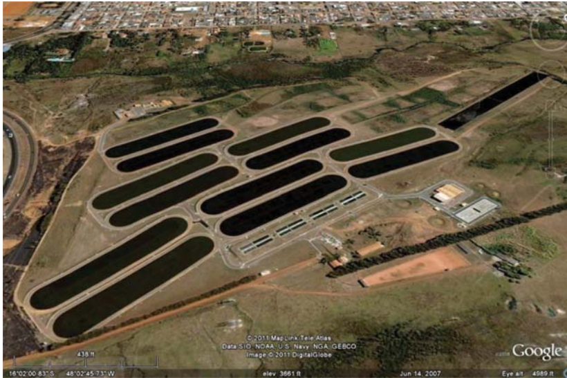
Figure 1.89 A satellite photo of the alagado treatment plant in Brasilia, Brazil, consisting of UASB followed by lagoons followed by overland flow
