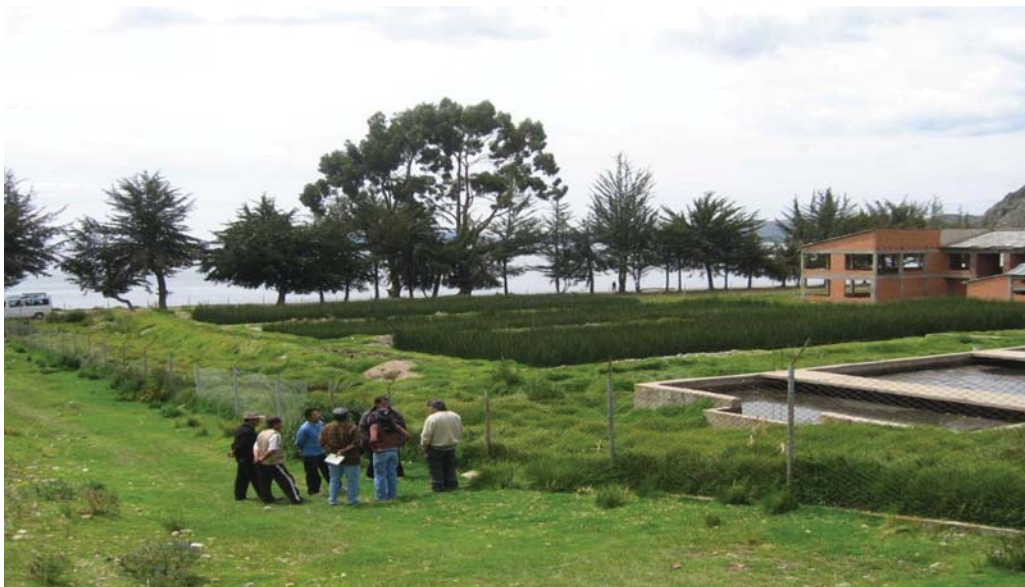
Figure 1.35 Photo of a constructed wetland plant in Copacabana, Bolivia
