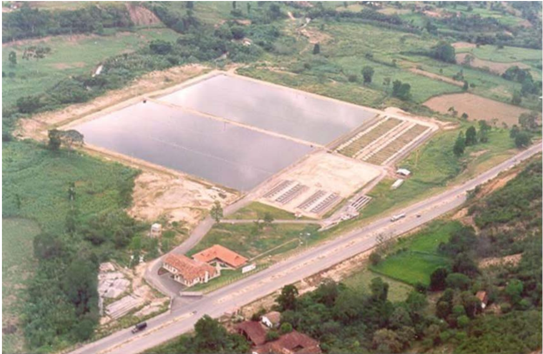
Figure 1.61 Air photo of the Rio Frio treatment plant in Bucaramanga, Colombia
