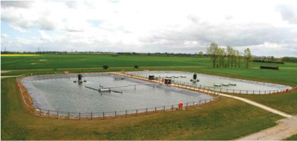
Figure 1.18 A facultative lagoons plant of Sutton St. James, England, with mixers and air injection systems (Courtesy Gurney Environmental)
