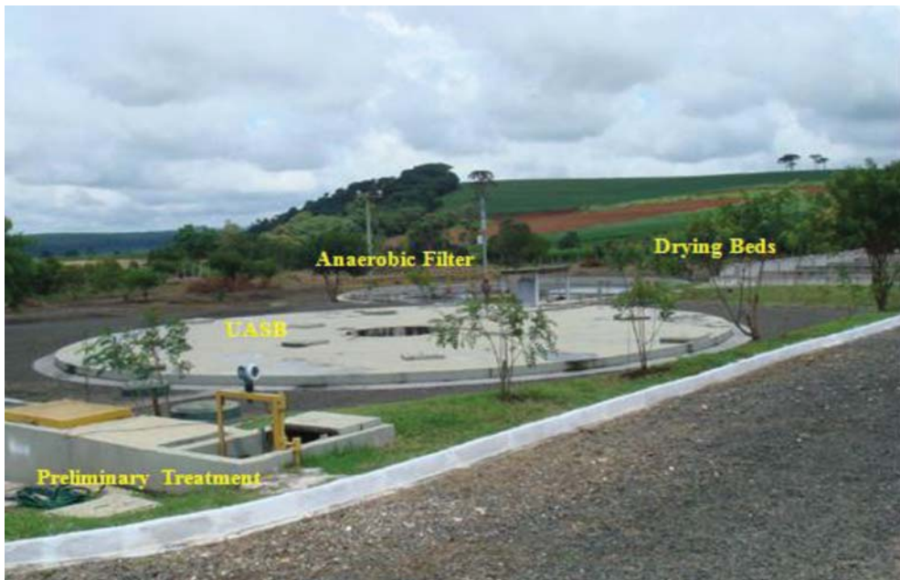
Figure 1.65 UASB reactor followed by anaerobic filter in Tibagi, Parana, Brazil
