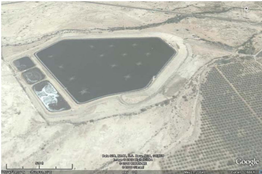
Figure 1.78 A satellite photo of the Og reservoir equipped with mixers which enable to increase the organic matter surface loading it is capable of handling
