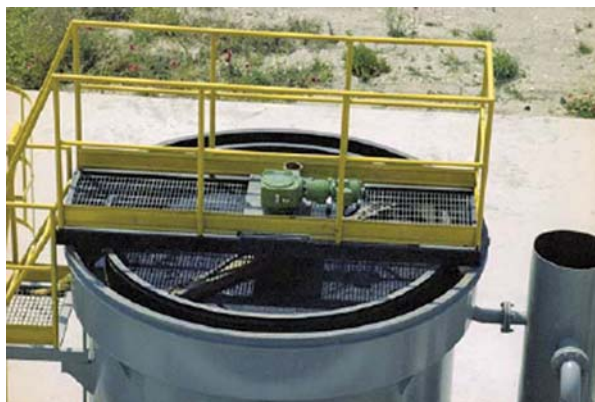
Figure 10.9 Photo of a typical DAF installation. [Source: http://www.sereco.it/share/img_prodotti/32img1.jpg ]
