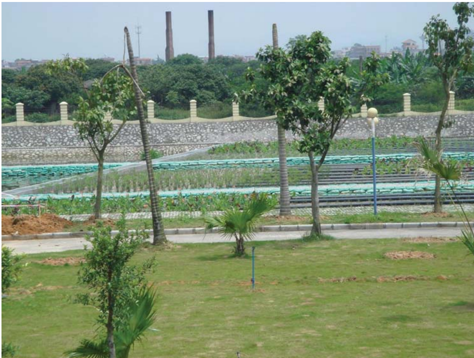
Figure 1.36 A constructed wetland unit used for polishing the effluent of an activated sludge plant serving a population of 120,000 in the province of Guandong in China
