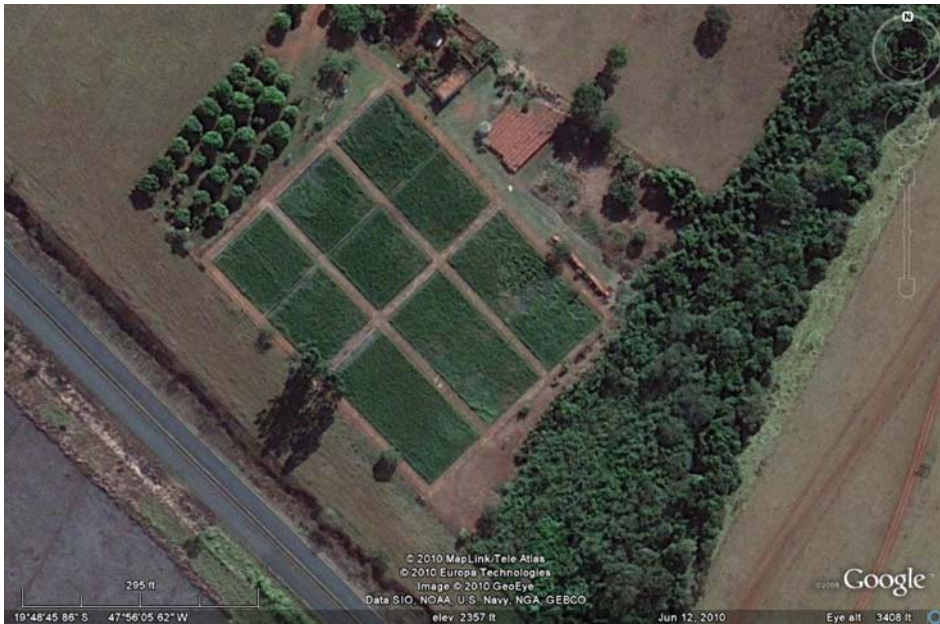
Figure 1.42 The capin overland flow system in the city of Uberaba, Brazil, serving a neighbourhood of the city with a population of 2,000
