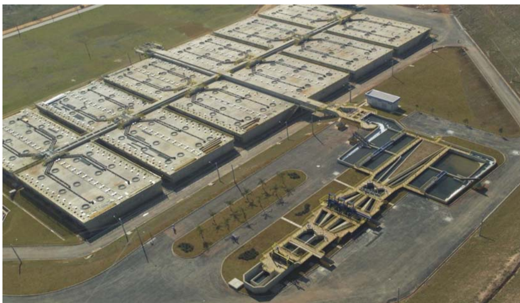
Figure 1.7 The Onca UASB treatment plant in the City Belo Horizonte, Brazil
