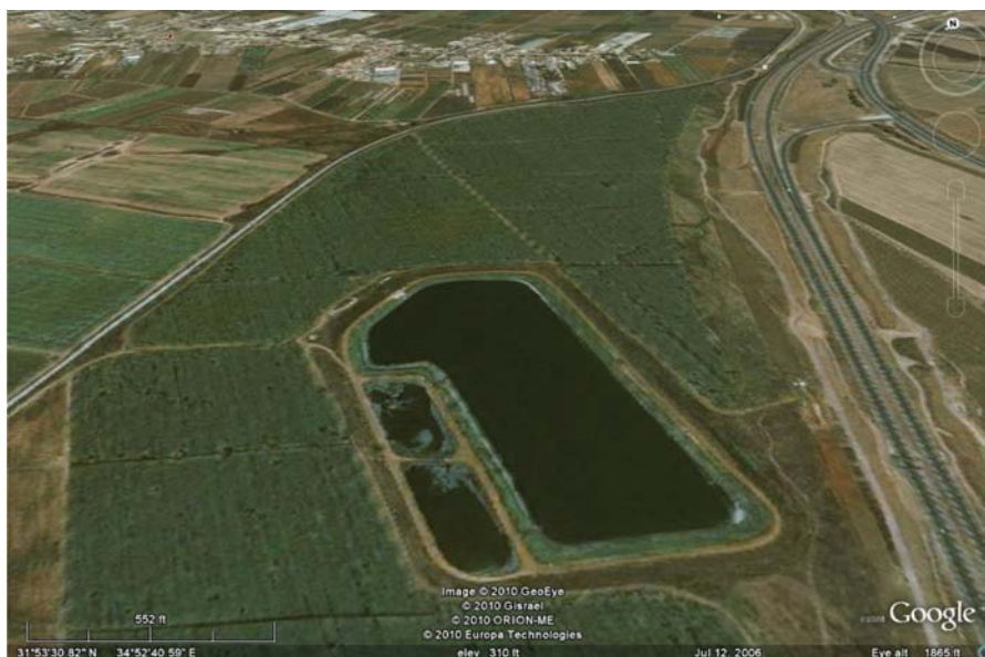
Figure 1.77 The Naan wastewater treatment system and stabilization reservoir
