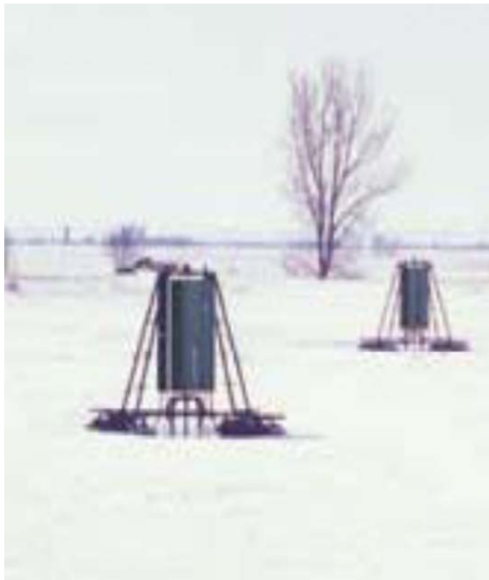
Figure 1.19 A facultative lagoon equipped with mixers functioning under severe winter conditions
