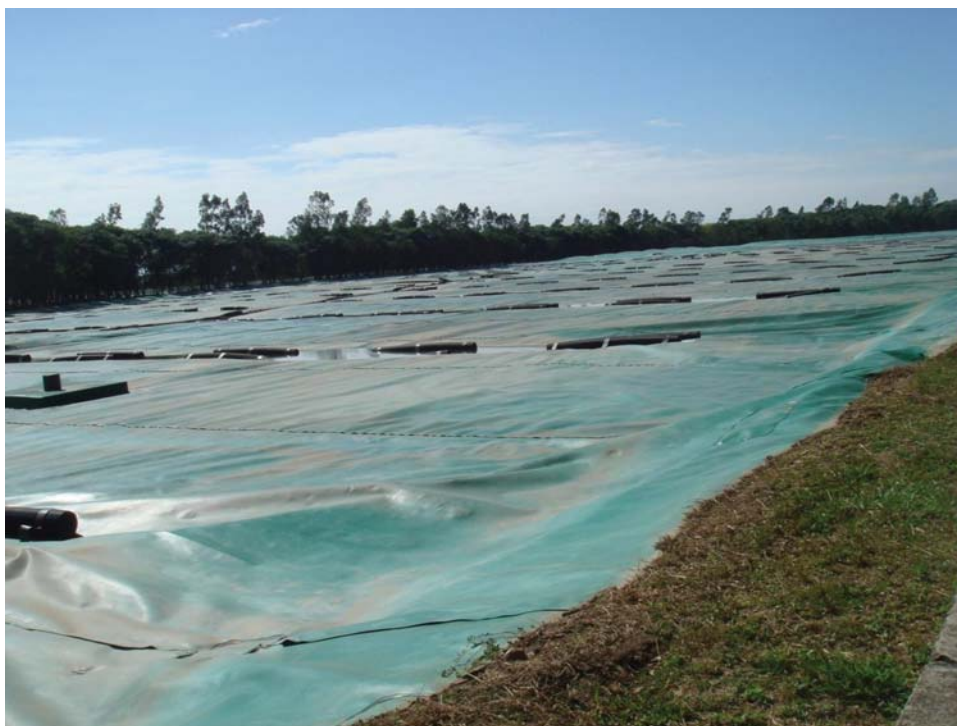
Figure 1.5 Covered anaerobic lagoons in a wastewater treatment plant in Santa Cruz, Bolivia
