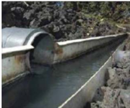
Figure 8.3 Inflow Distribution Structures [Source: WSP (2008)]
