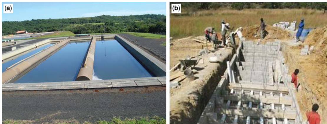
Figure 1.9 (a) A buried UASB tank under operation in the treatment plant of the City of Uberaba, Brazil. (b) Baffled reactor in Zambia (Source: http://www.germantoilet.org/en/projects/zambia/menu-sambia/progress.html )
