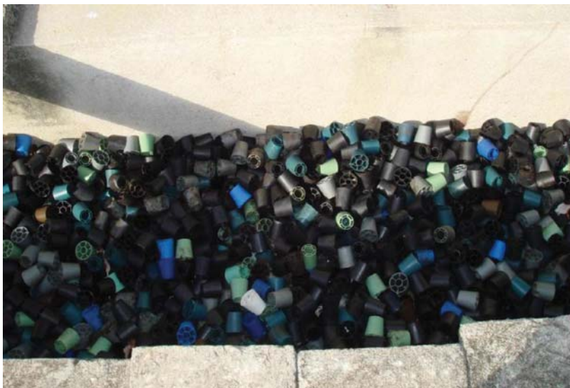
Figure 1.11 Anaerobic filter media composed of plastic material shapes with a large surface area
