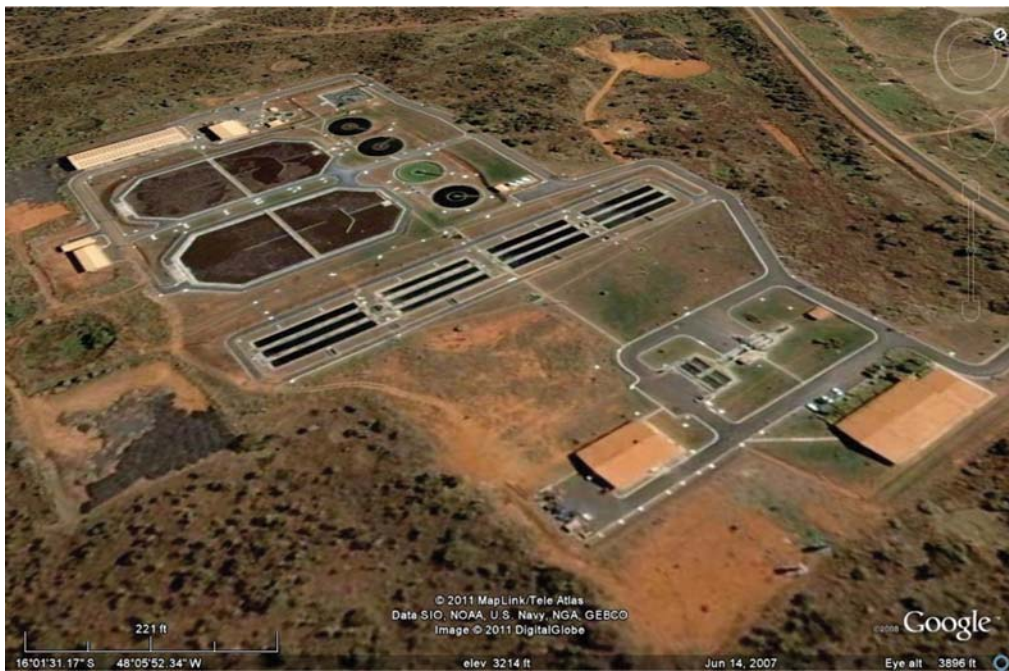
Figure 1.80 The Gama plant in Brasilia, Brazil, based on UASB followed by activated sludge, which does not constitute an appropriate technology process
