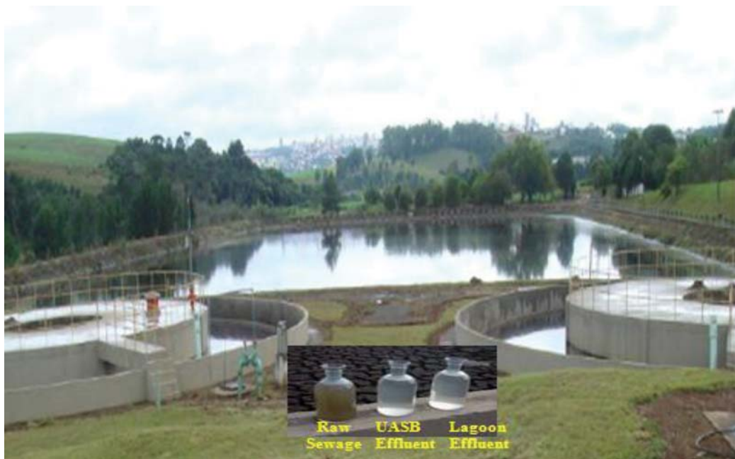
Figure 1.62 UASB reactors followed by a facultative lagoon in Ronda, Ponta Grossa, Parana, Brazil
