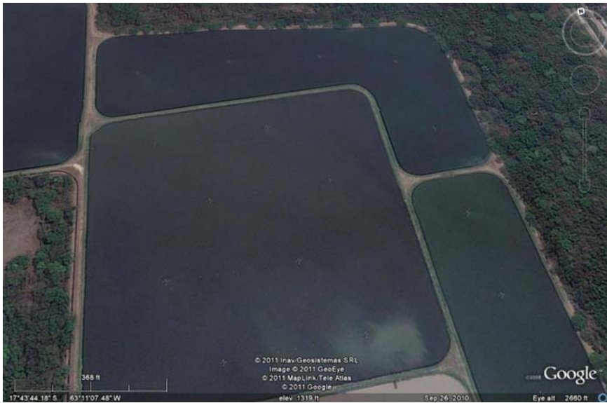
Figure 1.55 Mixers in the facultative lagoon of plant N2 after its upgrade
