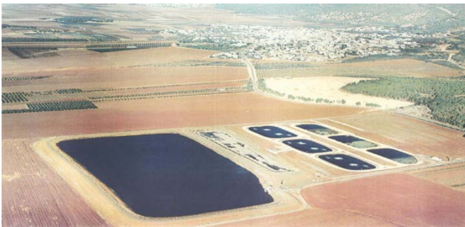
Figure 1.74 The wastewater treatment system and stabilization reservoir of the City of Nazareth—Photo taken in the 1980s
