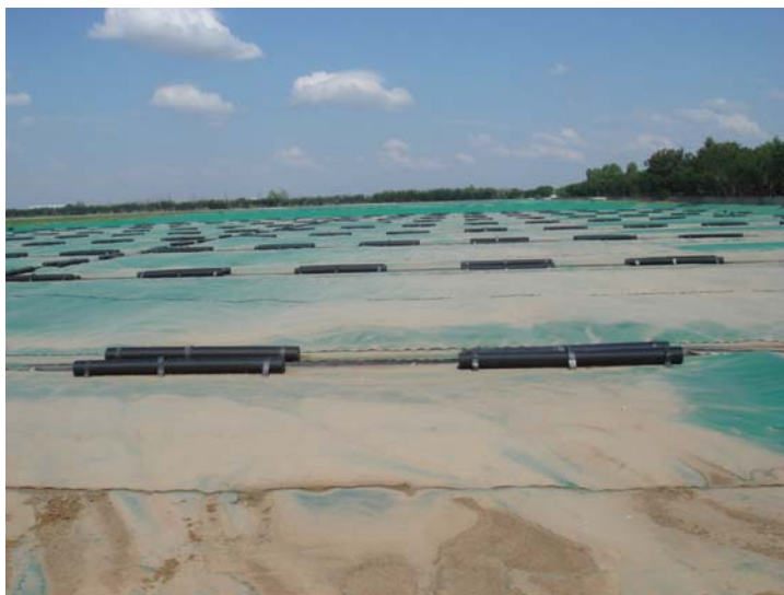
Figure 5.2 A covered anaerobic lagoon
