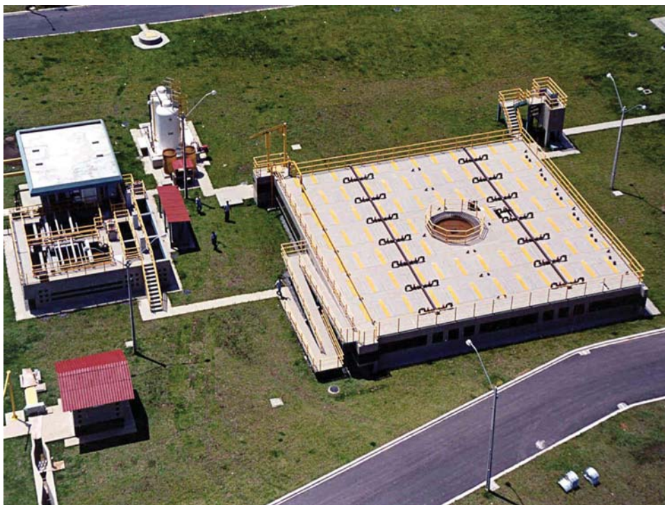
Figure 1.71 The treatment plant Sao Jorge in the City of Almirante Tamandare in the state of Parana, Brazil, based on UASB followed by dissolved air flotation followed by UV disinfection
