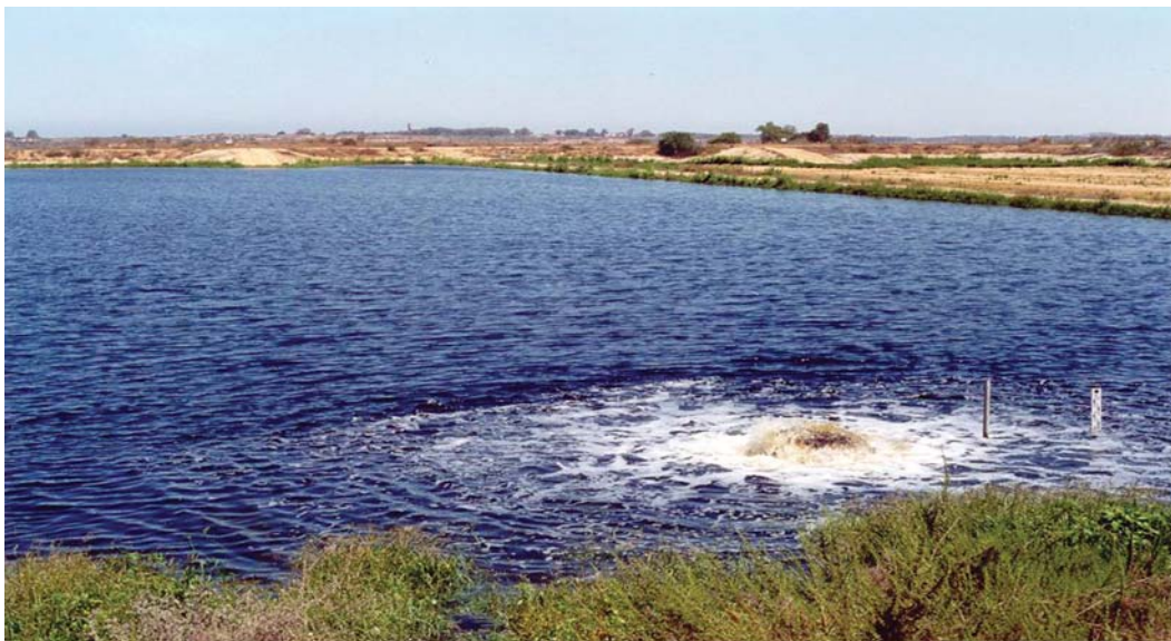
Figure 1.45 Photo of an infiltration basin after its inundation with effluent, initiating the infiltration process
