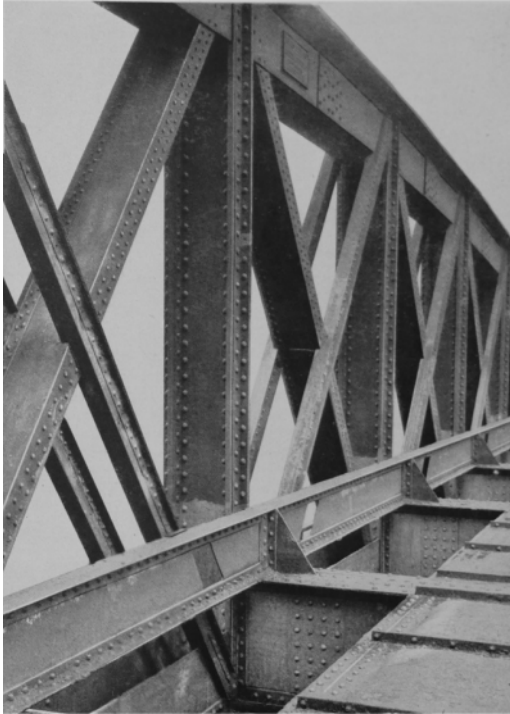
Figure 7. Repaired beam of the J-F Lépine bridge.
