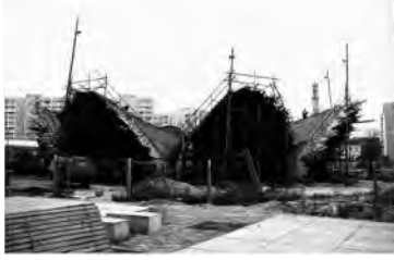
Figure 27. Scaffolding, 1982–1983. Mütter Archive of Wismar University.
