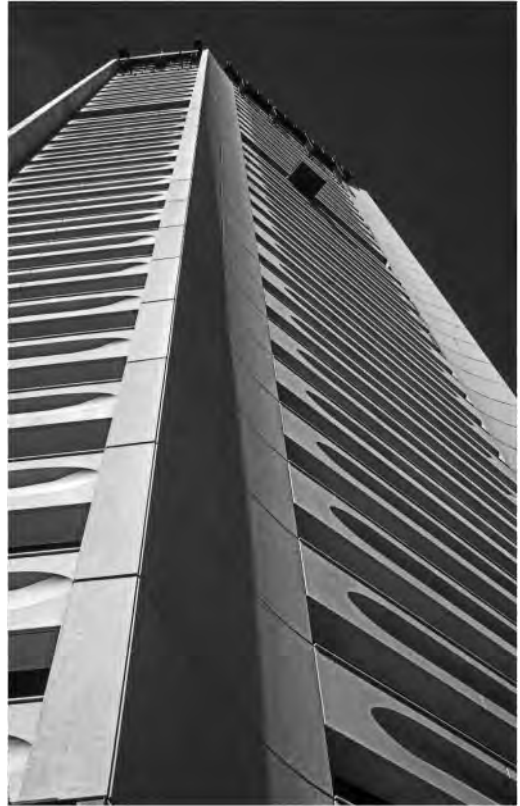
Figure 4. MLC Tower – Nervi's column profiles and beam-spandrels (cropped). © Penelope Seidler (photographer Harry Seidler).
