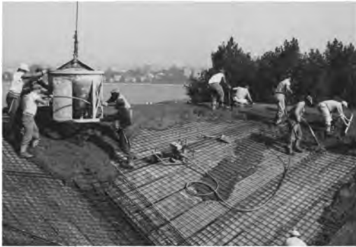
Figure 8. Construction process of the inverted umbrellas for the roof of the library building for the Hunter College, Bronx, New York, USA, 1958. Wire Reinforcement Institute.
