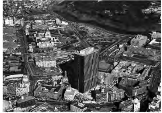
Figure 1. Kasumigaseki Building construction.
