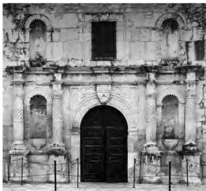
Figure 4. San Antonio façade (photo by the authors).
