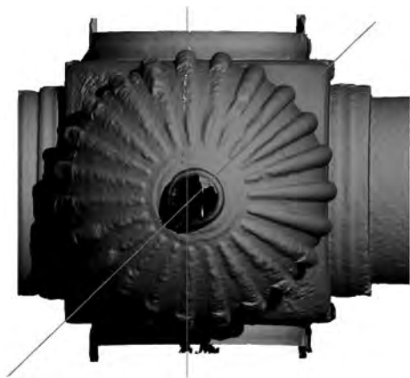
Figure 7. A rendering view of one scalloped dome from the three-dimensional survey (L. Repola UniSOB workshop).
