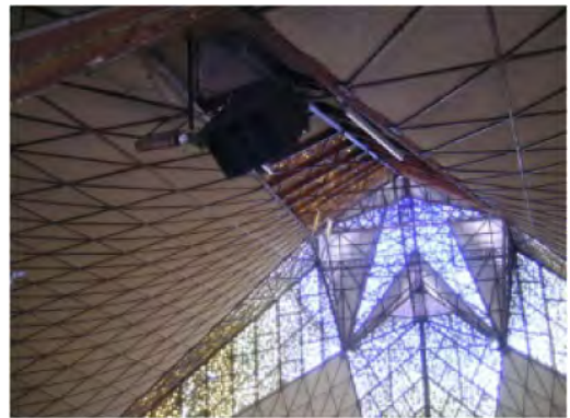
Figure 17. View of the bars forming the cover (Image Moisés Escárcega).
