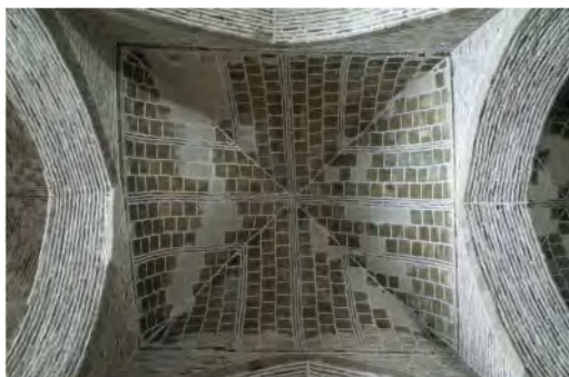
Figure 3. View of one of the timbrel vaults of the Friday Prayer Mosque of Isfahan.
