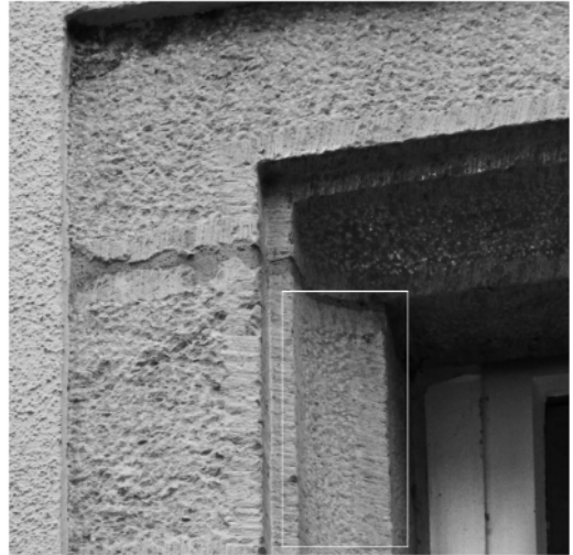
Figure 9. Solothurn, window with concavely curved soffits in Judengasse 5, 16th century. (author 2020).
