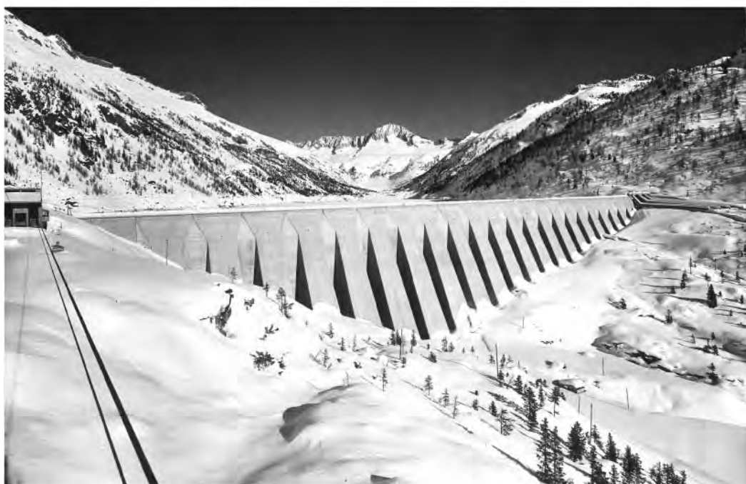
Figure 4. The hollow gravity “Marcello type” dam at Malga Bissina on the Upper Chiese River, 1955–57. View from the valley, in construction and completed (SIXXIdata: Claudio Marcello Private Archive).
