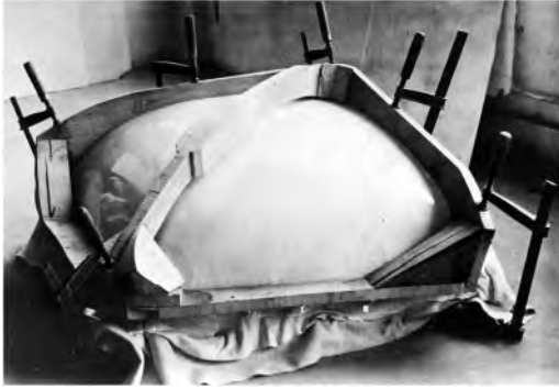
Figure 1. Forming of a strongly bent acrylic glass sheet for an omnibus window on a steel mold covered with cloth and a wooden pressure frame in the 1950s. Measurements of the window sheet: 1100 x 1100 x 5 mm, weight 7 kg (Röhms & Haas GmbH (ed.) 1965, 15).
