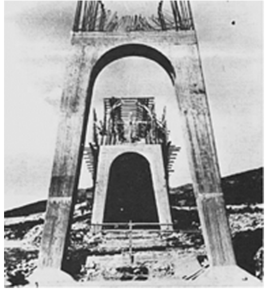
Figure 5. The piers in construction (Archivio Storico Enel).
