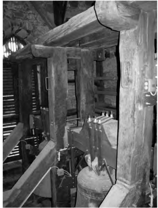
Figure 7. Kahla, St Margareten, bell frame, 1495, queen post construction. Photo: Iris Engelmann 2012/VG Bild.
