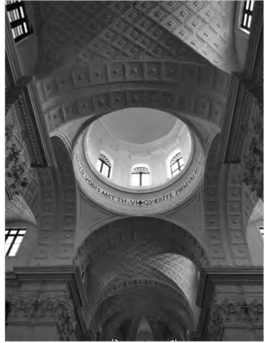
Figure 9. View of the vaults with sophisticated plaster coffers in St. Cajetan (Old Goa).
