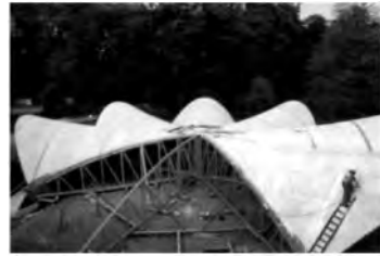
Figure 21. Precast segments lifted by crane and assembled into position, ca. 1976.
