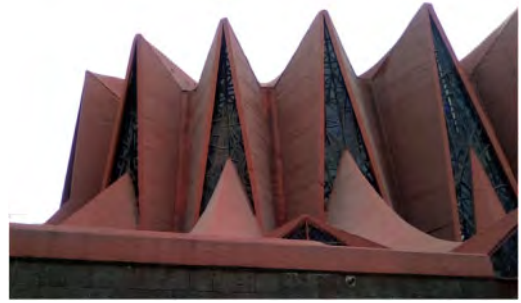
Figure 7. Visible outside the hyperbolic paraboloids of the chancel are the hyperbolic paraboloid that form the pillars of the cover and the radially arranged hyperbolic paraboloid (Image by the authors).
