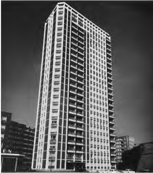
Figure 6. Tower of the Centro Romana district. Source: ACS, SGI collection, folder 4091–105, Photographic archive.
