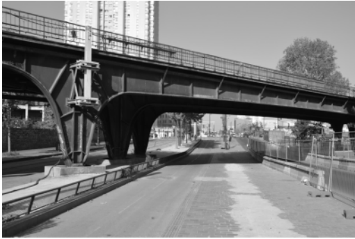
Figure 3. View of the bridge over the Boulevard Ney, photo taken by S. Sire, August 2020.
