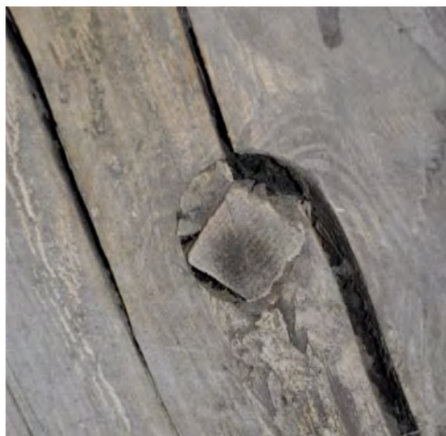
Figure 4. Toruń, parish church of St John, the roof structure over the north aisle, an opening in which there is a wedge and plated bands, which attests to the rafting of wood.
