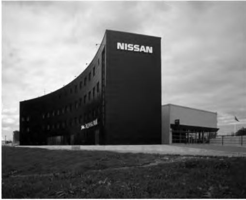
Figure 5. Nissan Centre in Tallinn.
