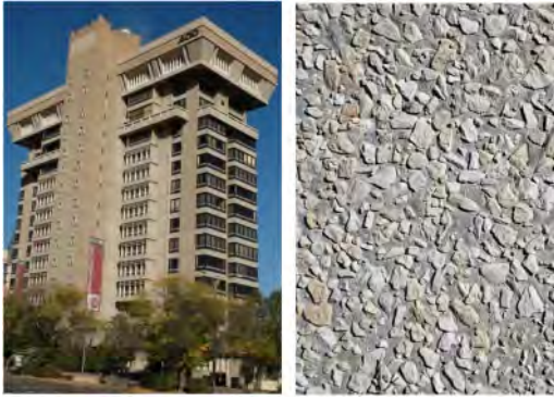
Figure 6(left) and 7(right). Pet Milk building, and exposed limestone aggregate. (photo credit: author).
