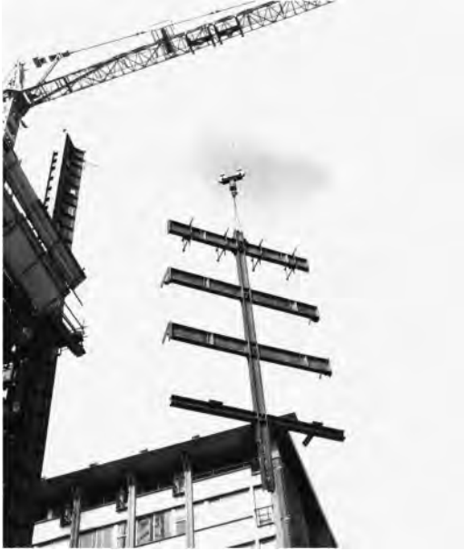
Figure 3. Humanities faculty of the University of Turin during construction, 1965–1966 (A. Goldstein Bolocan Private Archive).
