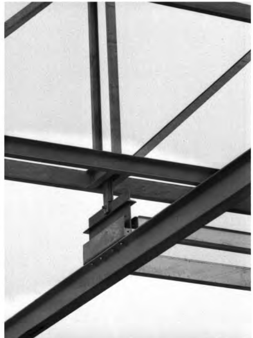
Figure 10. A couple of steel trusses and the sequence of underlying transversal beams (Courtesy of Franco Sargiani).
