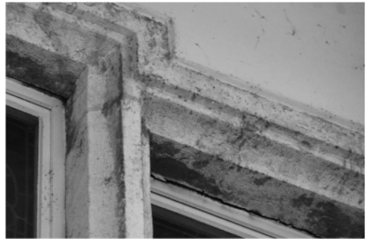
Figure 10. Window jamb in Friedhofsplatz 14, mid-17th century. (author 2020).
