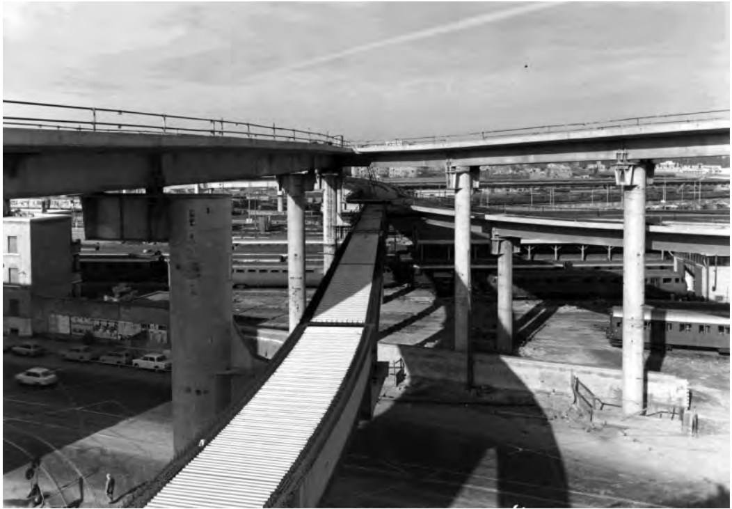
Figure 9. Rome flying road during the construction, 1969–1972 (Ansaldo Foundation Historical Archive).
