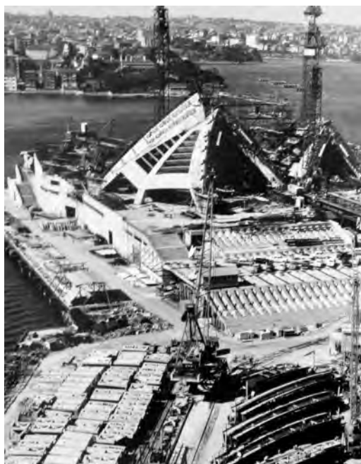
Figure 1. The casting yard from the roof of Unilever House. NSW Archives and Records NRS:4_7927 (photographer unknown).
