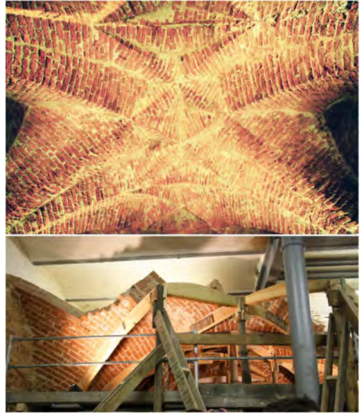
Figure 8. Above: Diamond vault at Trebsen Castle (Germany). Below: experience of reproducing it on a 1:1 scale in a workshop led by Professor David Wendland at the University of Dresden in the year 2012 (photographs by Enrique Rabasa).
