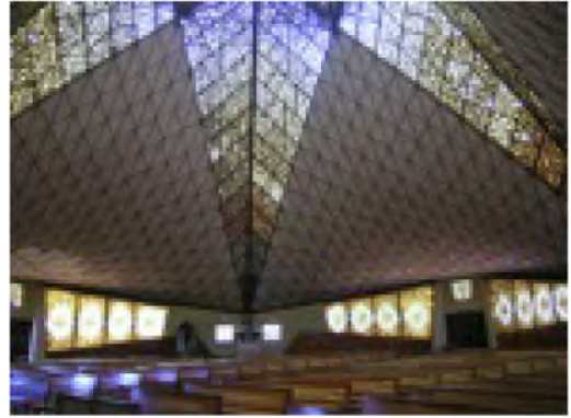
Figure 15. Interior of the church. The two paraboloid sections join only at the concrete support (Image Moisés Escárcega).
