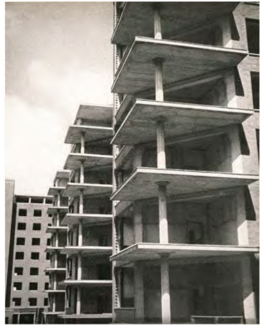
Figure 2. The solariums, all located on corners to take advantage of southern sunlight, are differentiated by using a reinforced concrete cantilever square-plan slab supported by three pillars. Archivo Torroja, CEHOPU-CEDEX, I-ETM-095-09/C.
