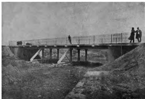
Figure 5. A road bridge in Trituznyj Chutor, erected in 1902 (Černomorskoe Stroitel'noe Obščestvo 1906).
