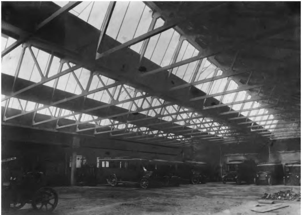
Figure 3. 1920, L. Santarella, Garage Fossati, Biella. Interior view of the roofing system (A. Bologna, private archive).
