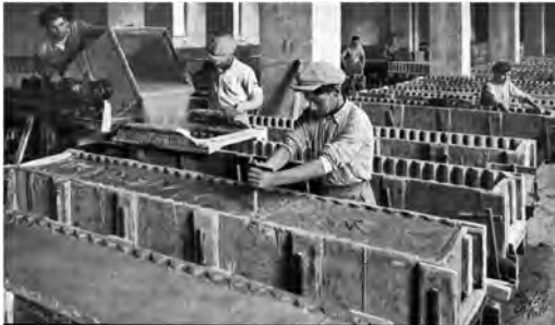
Figure 2. Cellular concrete blocks under production in Porto Hospital (Revista Técnica no. 189, 1949).
