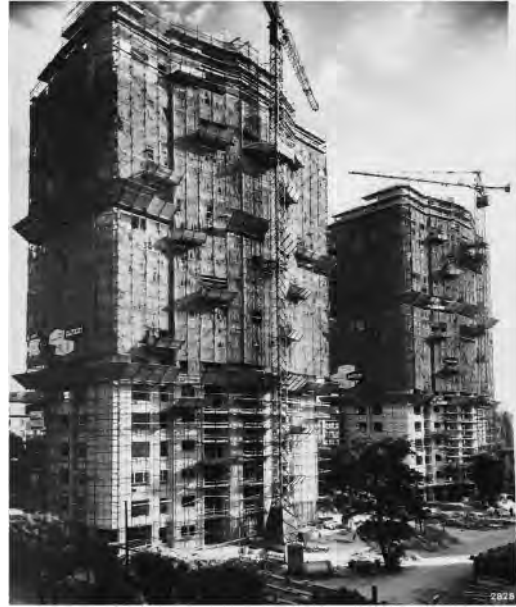
Figure 4. Towers of the Monti-Pagano district under construction. Source: ACS, SGI collection, folder 4091-265, Photographic archive.
