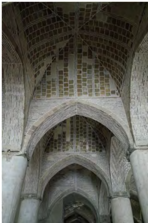
Figure 1. Timbered vaults in the Friday Prayer Mosque of Isfahan.
