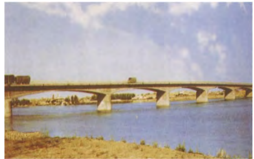
Figure 1. The Bridge over the Euphrates in Fallujah, Iraq (1964–67). Source: Ačić et al., 2012, p.148.
