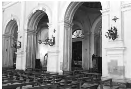
Figure 6. Surveys on arches and pillars by plaster removal.
