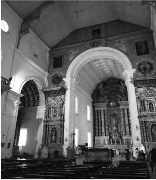
Figure 1. Bom Gesù, Jesuit church in Old Goa. Prototype church with crossing trellis vault in the chancel.
