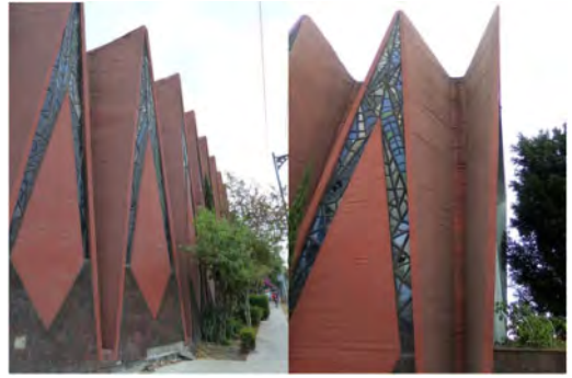
Figure 12. Exterior of the building showing the arrangement of the supports for the different sections. They consist of two ruled surfaces that increase in width from bottom to top (Image of the authors).
