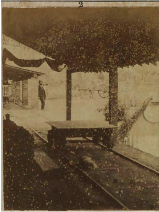
Figure 7. Inclined plane on which the steam wagon that transported clay to the machines functioned. Date: 1869. Collection from the Brazilian National Library. Available at: http://acervo.bndigital.bn.br/sophia/index.asp?codigo_sophia=42171 . Accessed 26 November 2020.
