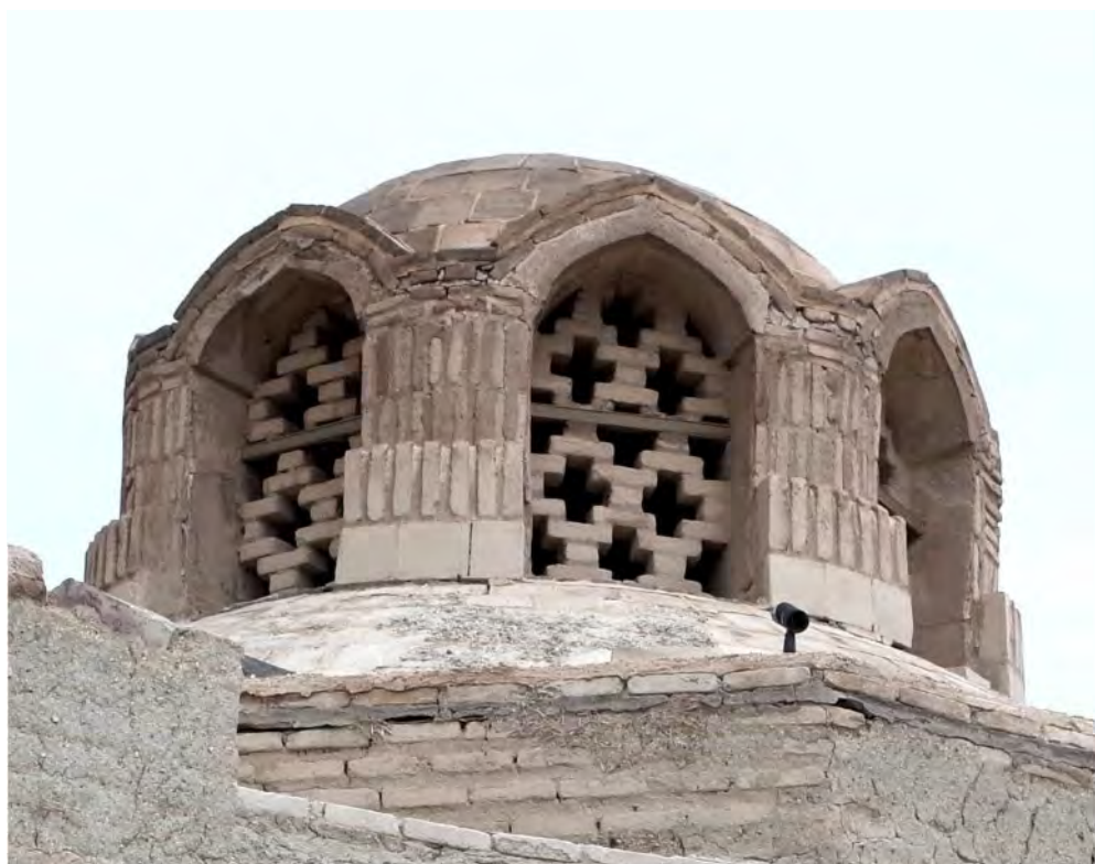
Figure 9. Lantern crowning a dome in Nain with small timbrel vaults over its windows.
