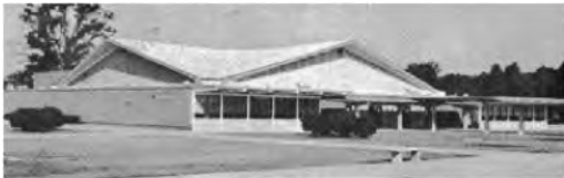
Figure 1. Gymnasium of the Henrico High School, Virginia, a gabled-type hypar shell structure similar to the Tucker High School (Students clear...1970).
