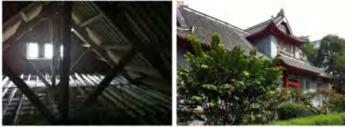
Figure 8. In the architecture of WCUU, there was no raising and depression in the roof truss (left), making it heavy and unwieldy (right). Source: photo by the author.
