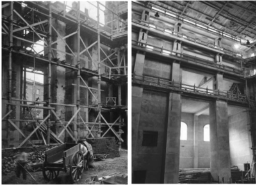
Figure 13, 14. The reinforced masonry pillars. –The pillars with the Vierendeel shape. Donati & Zanichelli Company's private archive.
