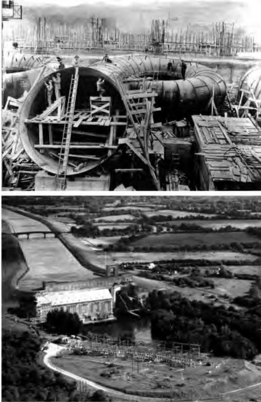
Figure 4. Penstock Ardnacrusha hydroelectric station (courtesy ESB Archives).
