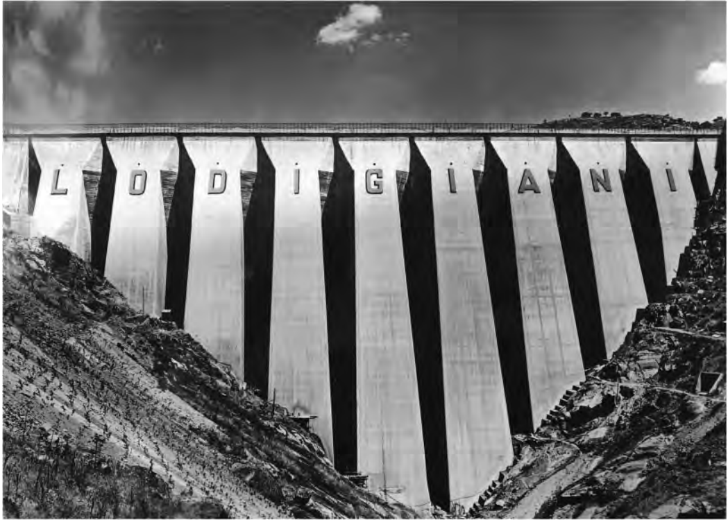
Figure 5. The hollow gravity “Marcello type” dam at Ancipa on the Troina River, 1949–52. View from the valley (SIXXIdata: Claudio Marcello Private Archive).
