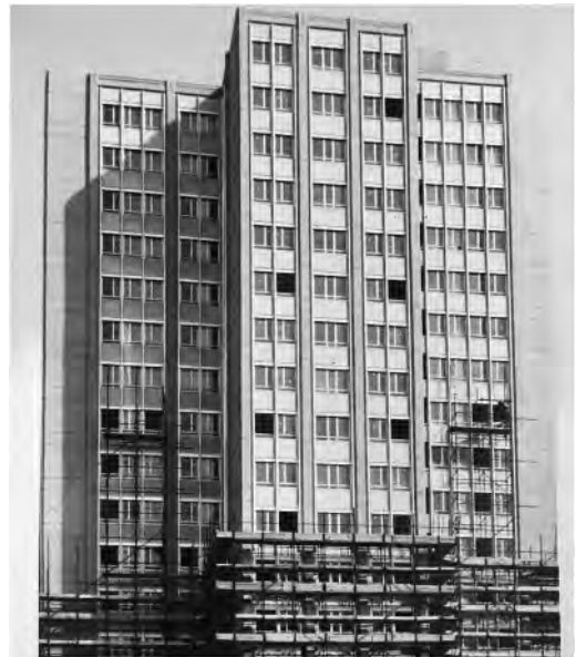
Figure 12. Cantore Tower façade. Source: ACS, SGI collection, folder 4091–88, Photographic archive.
