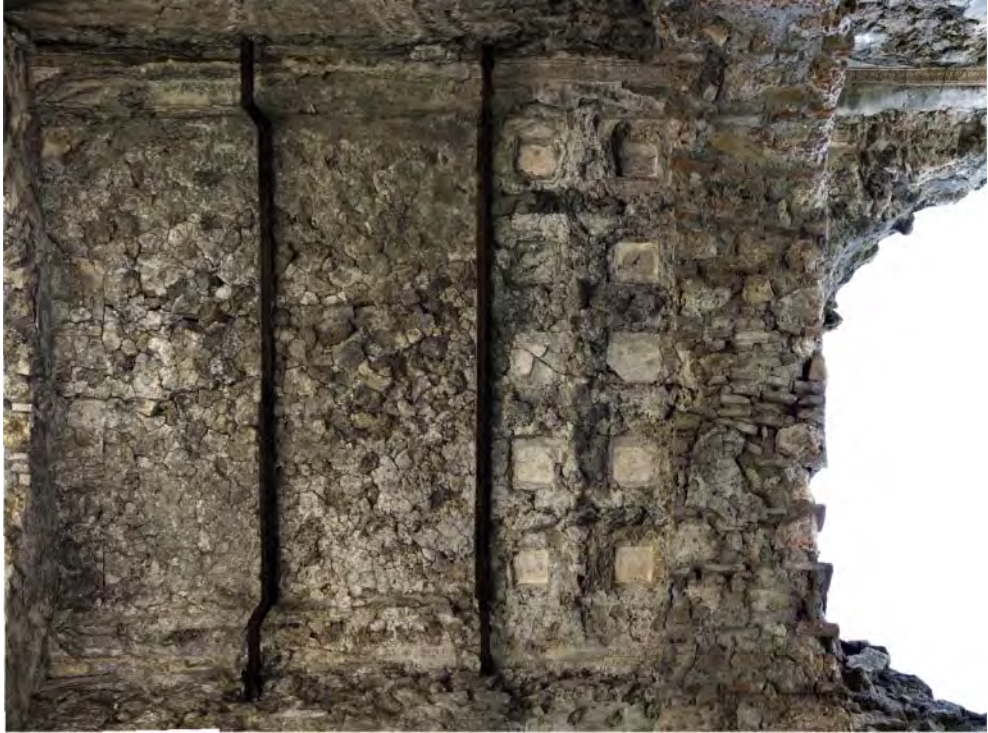
Figure 2. Orthophotograph of the concrete floor in area N°. 46, internal view (Thomas Crognier 2015).
