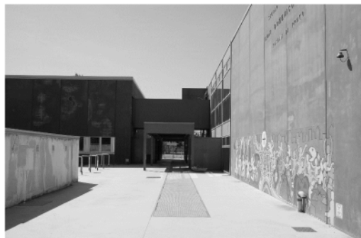
Figure 7. School in Pasion di Prato built with Valdadige system (Albani 2017).
