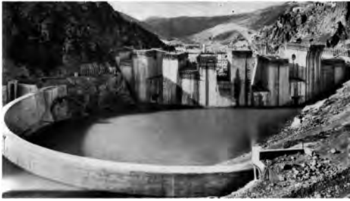
Figure 1. Bemposta dam under construction (MOP 1963, 25).
