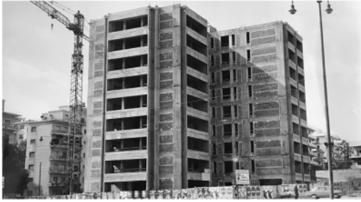
Figure 13. Sperlina Tower under construction. Source: ACS, SGI collection, folder 4091–148, Photographic archive.
