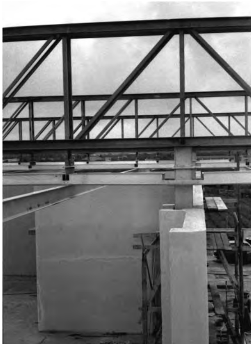
Figure 10. A couple of steel trusses and the sequence of underlying transversal beams (Courtesy of Franco Sargiani).
