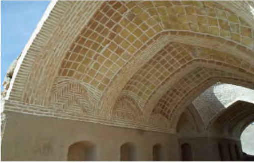
Figure 4. Timbrel vaults in the Yazd funerary complex.
