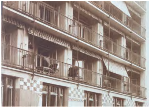
Figure 8. Photograph of the cantilever in front of the patients' rooms (source: Staatsarchiv Thurgau StATG 9'11, 10.4/0).
