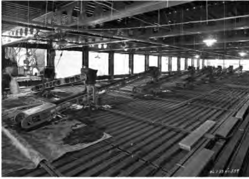
Figure 6. Concrete conveyors.
