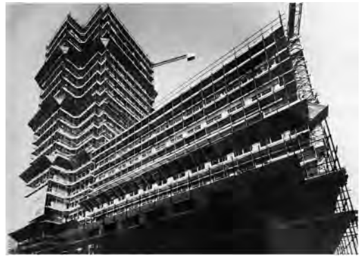
Figure 11. Cantore Tower site. Source: ACS, SGI collection, folder 4091–88, Photographic archive.
