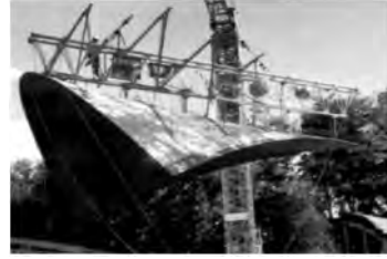
Figure 20. Precast segments lifted by crane and assembled into position, ca. 1976.
