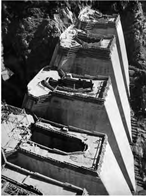
Figure 3. (On the left) Hollow elements of a gravity “Marcello type” dam. Ancipa Dam on the Troina River, 1949–52; (on the right) Hollow gravity “Marcello type”, Bau Muggerris Dam for the Upper Flumendosa River plants, 1948–49. View from valley (SIXXIdata: Claudio Marcello Private Archive).
