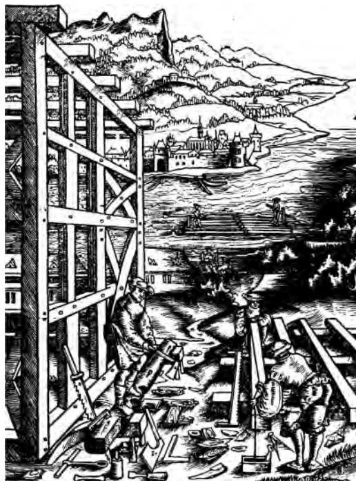
Figure 11. A carpentry yard with a carpenter standing on a log and making transverse cuts with an axe, 1531, cf. Binding et al. 1989.
