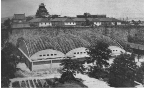
Figure 8. Three shells of the Osaka Castle Shooting Range (Osaka Construction Department of the Japan Self-Defense Force 1956).
