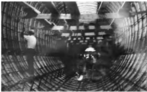
Figure 11. Interior of the conduit before the casting (ASE).
