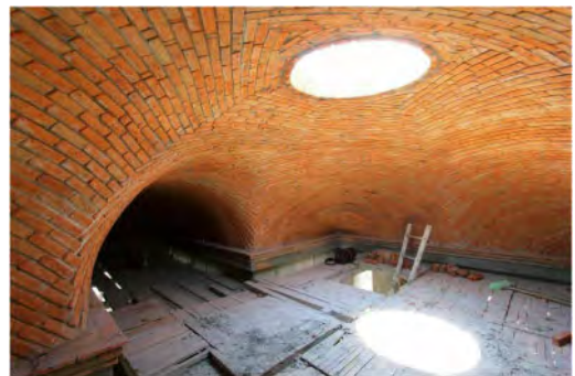
Figure 12. Current Mexican vault built by Andrés Flores Castañeda, 2020 (photograph by Andrés Flores).
