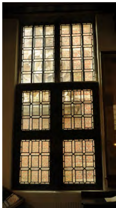
Figure 1. Cross-window in the Gulden Passer, situation after 20th-century reconstruction.
