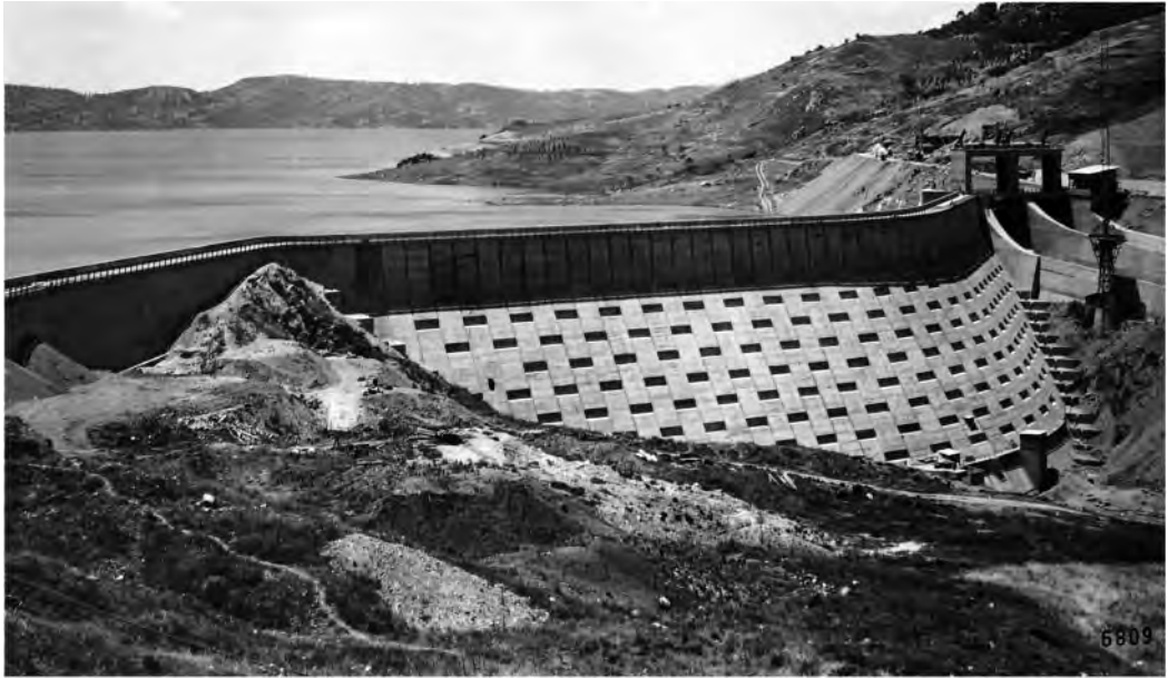
Figure 8. Pozzillo Dam on the Salso River in concrete blocks, 1956–58. View from the valley of the completed dam (SIXXIdata: Claudio Marcello Private Archive).
