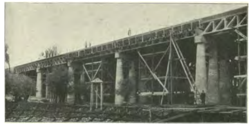
Figure 8. The construction site of the bridge near Černigov (von Emperger 1911).
