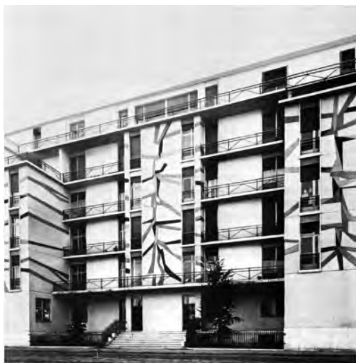
Figure 2. Building in via Gorizia by M. Zanuso, 1950–51. Source: Bottoni 1954.
