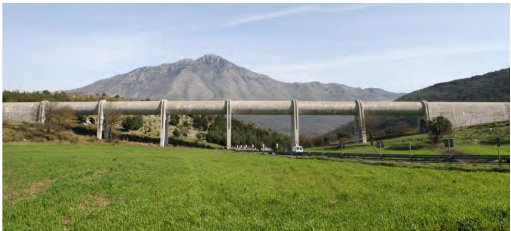
Figure 3. Adriano Galli, aqueduct over the Casilina in Mignano Monte Lungo, Campania, 1952–4 (source: the authors).
