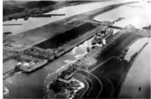
Figure 1. Overview of the Northern Lock, 1950s-1960s (Image courtesy Beeldbank Rijkswaterstaat).
