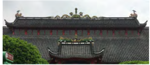
Figure 10. Exterior of detailed decoration of clay plastering on the “Chinese roof” of West China Union University Library Source: photo by the author.
