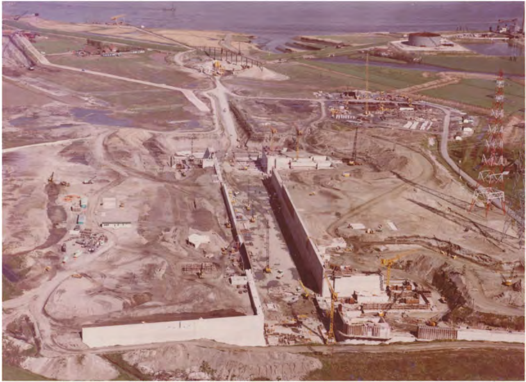
Figure 4. Kallo lock Antwerp, circa 1975. Van Laere is responsible for the complete execution, with its own techniques and resources. At the back, the river Scheldt is clearly visible, with Van Laere's very own loading quay, its own concrete plant, and its own infrastructure network, techniques and materials. (Guido Coolens).
