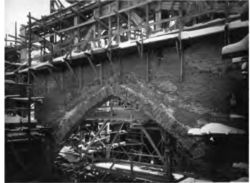
Figure 15. The consolidation and caging works of the wall. Donati & Zanichelli Company's private archive.
