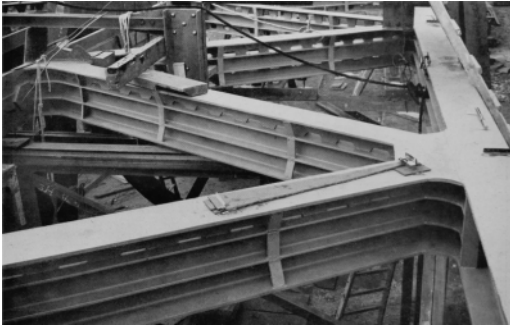
Figure 6. Load test on the truss of the Joncherolles bridge.
