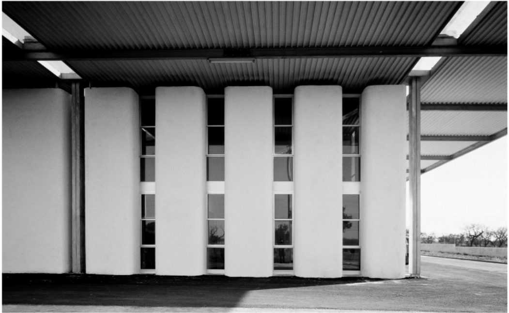
Figure 11. The building façade corresponding to the offices: the detachment between envelope and roof highlights the different nature of the building components (Courtesy of Franco Sargiani).
