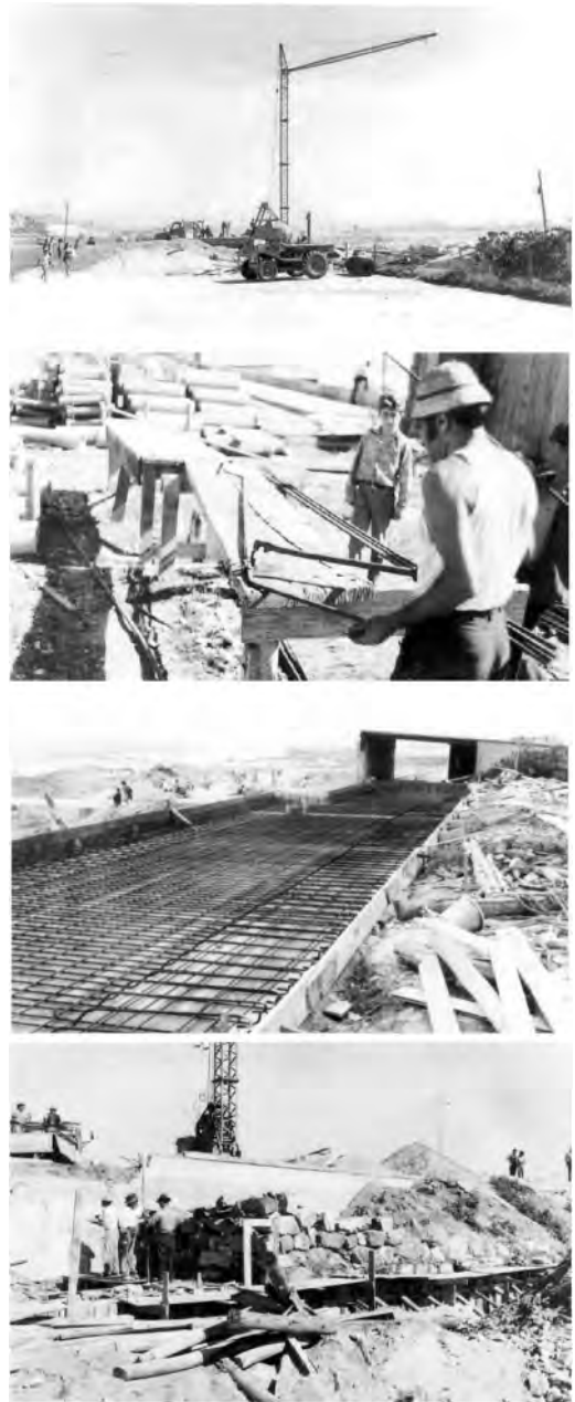
Figure 13. Ocean swimming pool, building site, 1971 (Mota 1972; Centro de Documentação da FAUP).
