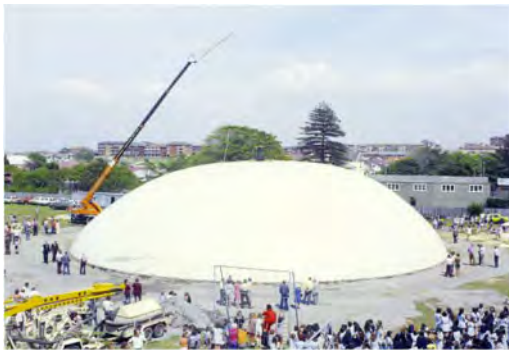
Figure 11. Inflation of a Binishell.
