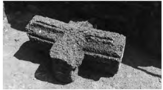
Figure 5. Crossing of a crossing trellis vault. Church St. Augustine, Old Goa.
