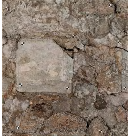
Figure 6. Detail of a coffer with a mortar (without terracotta) “tile” (Hélène Dessales 2015).
