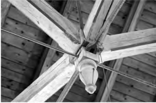
Figure 6. Cast-iron shoe at the bottom of the queen rod in the riding hall of Thun (Russnaik 2020).
