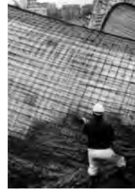
Figure 29. Gunite spraying, 1982–1983. Mütter Archive of Wismar University.
