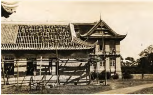
Figure 6. Small tiles being laid for the “Chinese roof” project at West China Union University Source: Archives of the United Board for Christian Higher Education in Asia, ubc416-5203. Credit: Digital Collection: Divinity Library Photographs, Yale Divinity Library.
