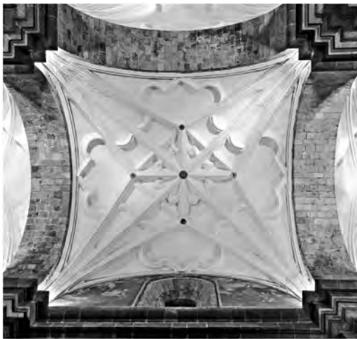
Figure 7. Cathedral of Cusco. A cross vault in the aisle, bottom view, current state after restoration (in Flores 2013).
