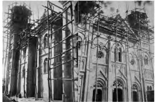
Figure 6. Xinjiang Cathedral, masons at work on the south-east spired tower, 1937 (© Het Utrechts Archief, 1224, 291/46–47).
