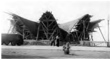
Figure 10. Mirvari Café under construction, ca. 1960.
