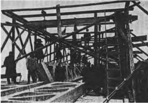
Figure 9. Setting up the truss girder (Hess 1911).
