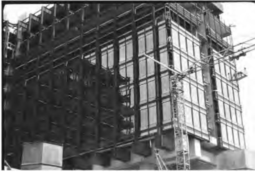
Figure 2. Placement of glazing on a wing of the former headquarters of La Royale Belge in Watermael-Boitsfort. Source: the private archives of Benoît Berdoux.
