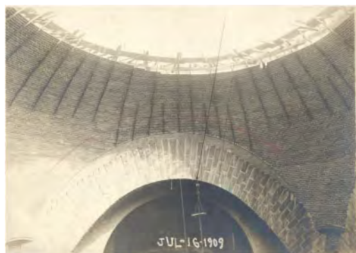
Figure 8. Construction progress photo of the dome at the crossing of St. John the Divine, July 16, 1909. Note the vertical form guides placed on the completed portion of the dome. Image provided by Episcopal Diocese of New York.
