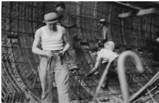
Figure 12. Carpenters working on the reinforcement (ASE).
