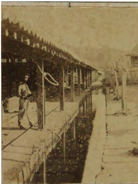
Figure 8. Houses where bricks were dried, water canal and pressure pump to wet bricks. Date: 1869. Collection from the Brazilian National Library. Available at: http://acervo.bndigital.bn.br/sophia/index.asp?codigo_sophia=42172 . Accessed 26 November 2020.
