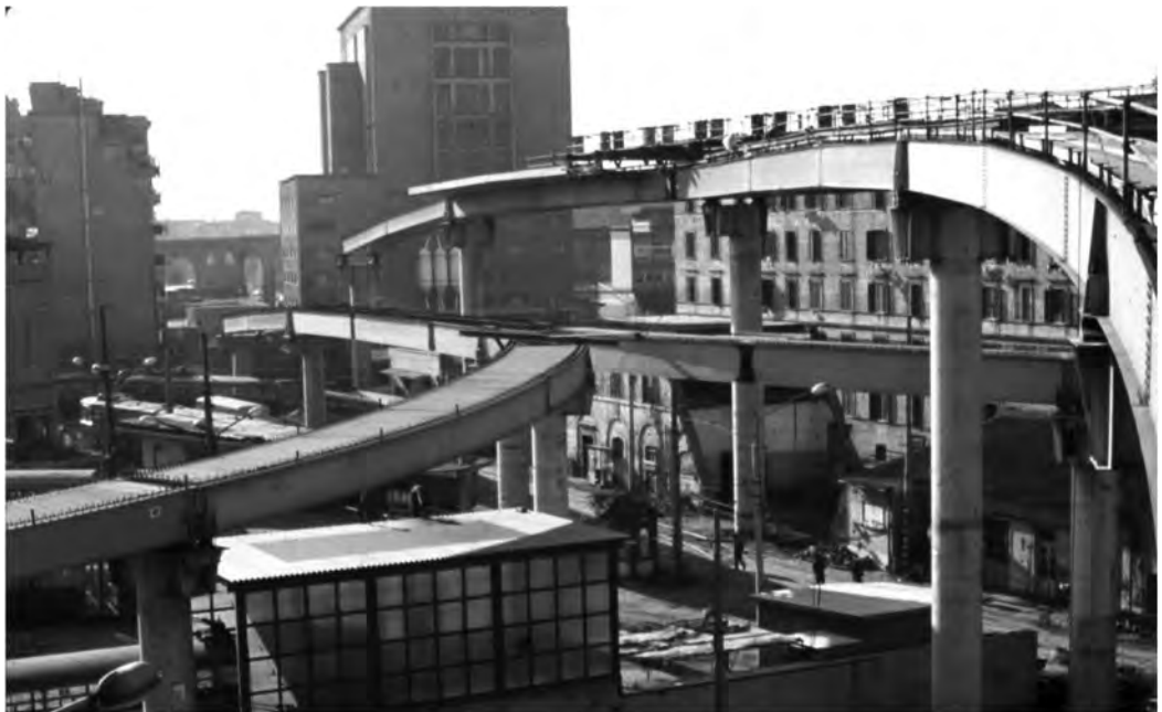
Figure 10. Rome flying road during the construction, 1969–1972 (Ansaldo Foundation Historical Archive).
