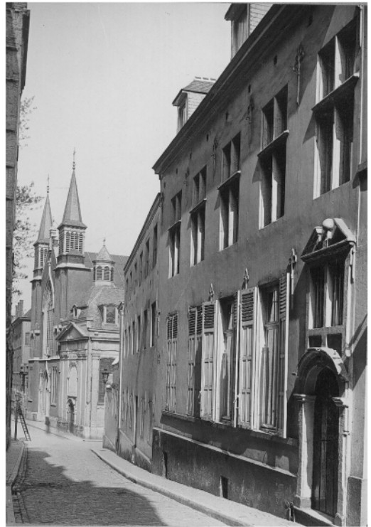
Figure 8. The door and window frame at Rue Terarken 4, depicted via a photographic campaign in 1907, were salvaged during the demolition of the street in 1910. Collection Comité d'Etudes du Vieux Bruxelles . © KIK-IRPA Brussels.
