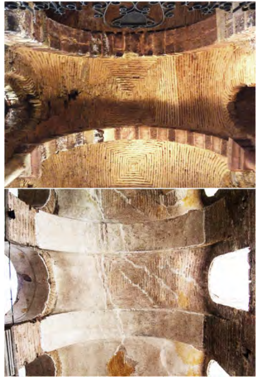
Figure 6. Above: Vaults of the pre-Absidian spaces of the church of the castle of Calatrava la Nueva (13th century). Below: vaults of Hagia Eirene in Constantinople (6th century). The similarity between the techniques is clear (photographs by Ignacio Javier Gil Crespo and Enrique Rabasa).
