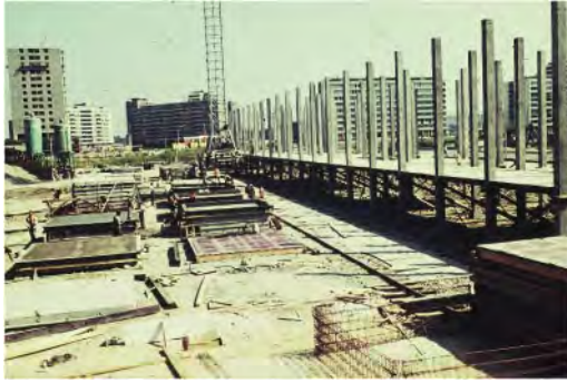
Figure 3. Experimental construction site of IMS Žeželj technology in Block 2 in New Belgrade, Serbia, ca. 1960. Source: Institute IMS archive.
