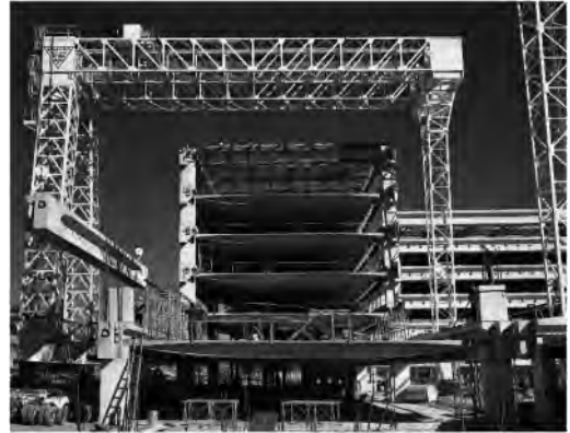
Figure 3. Implementation of the Nervi's "T" and "I" beams at the TGO building (today Edmund Barton Building), 1973. © Penelope Seidler (photographer Max Dupain).
