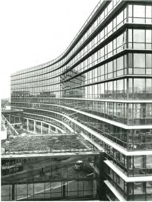
Figure 3. Façade of the tertiary building located at Square de Meeus n° 8 in Brussels. Source: private archives of Sophie Vantiegheem.
