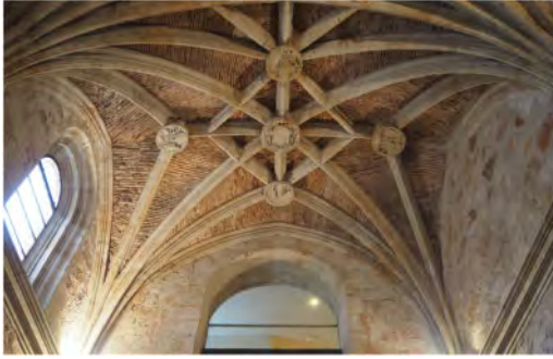
Figure 7. Vault of the Colegio de San Pelayo (University of Salamanca) showing the use of brick vaulting for the webbing (photograph by Enrique Rabasa).
