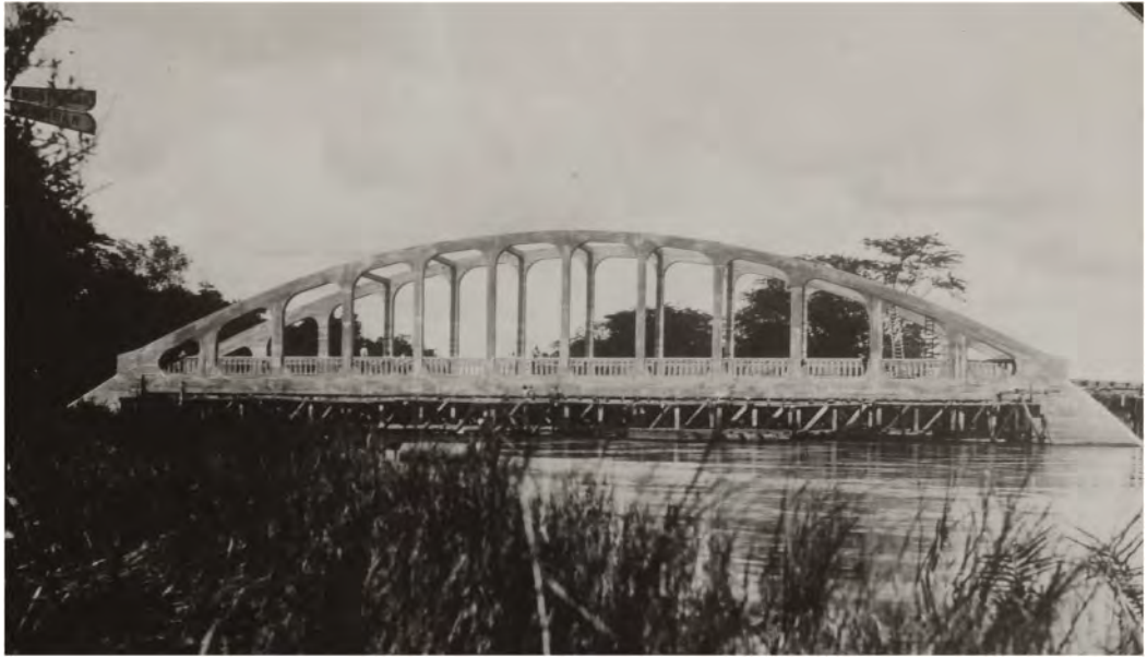
Figure 8. 48 m span concrete “Vierendeel” type road bridge built in 1931 over the Lufira River, still resting on its centre (Belgian State Archives).
