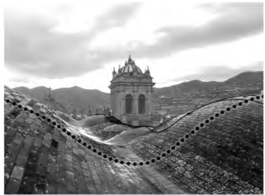
Figure 9. Cathedral of Cusco. The “flat roof” and the extrados of the vaults (the slope of the surface in evidence).
