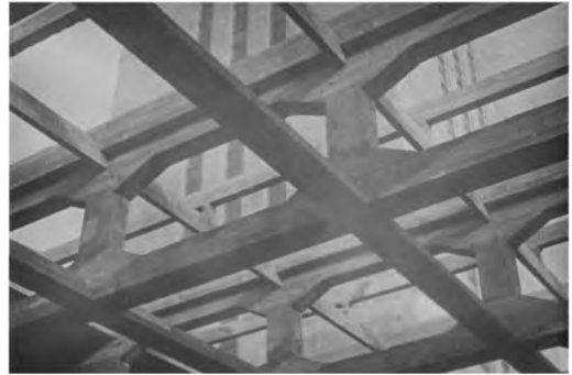
Figure 3. Detail of the Vierendeel trusses in the large reading room.
