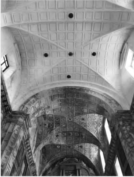
Figure 8. View of the vaults with the grid in relief carved in the chancel and in the first part of the nave in the St. Francis of Assis church (Old Goa).
