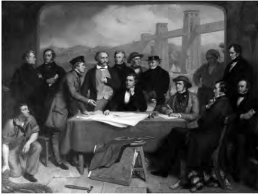
Figure 1. Robert Stephenson – Britannia Bridge (courtesy of the ICE).
