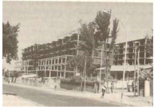
Figure 7. IMS Žeželj plant and the first building “Bole 100 AB” built using the system in Addis Ababa. Source: IMS '87, 277.
