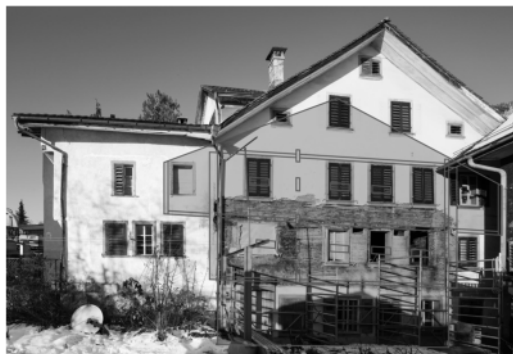
Figure 7. House Gütschweg 11, Schwyz, Canton Schwyz, Switzerland. The building before the investigations. Traced, the late medieval log construction from 1311, which was in large parts intact at the time of the survey (Gollnick & Frey 2016).
