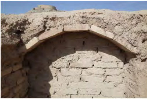
Figure 5. Segmental timbrel vault clad with adobe bricks.
