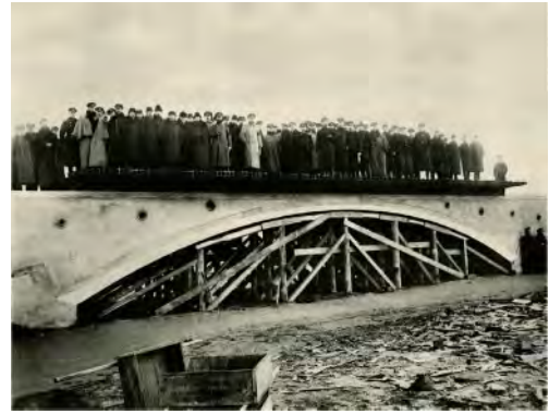
Figure 3. The official load tests that were held in Saint Petersburg in 1891 (Aktionernoe Obščestvo 190).
