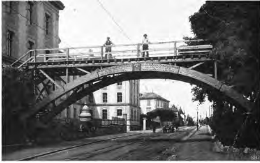
Figure 2. Footbridge built on the occasion of the National Agricultural Exhibition of 1910 in Lausanne, with a span of 27 m. The loading test was initiated and carried out by the SBB.
