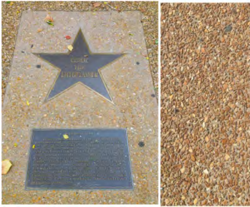
Figures 2(left) and 3(right). Delmar Boulevard Walk of Fame, detail photo of surface with exposed aggregate. (photo credit: author).
