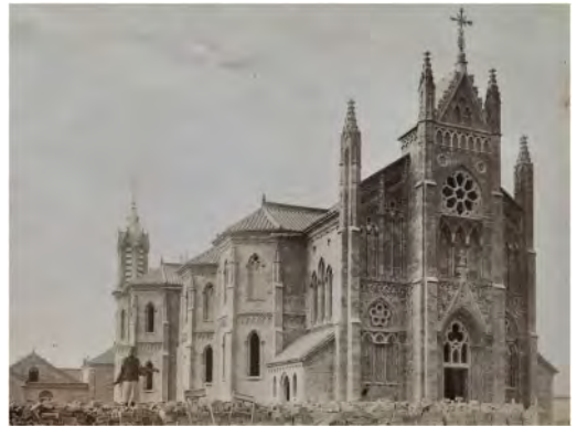
Figure 12. Lu'an Cathedral under construction, view from the south-west, 1903 (© Het Utrechts Archief, 1224, 289/4).
