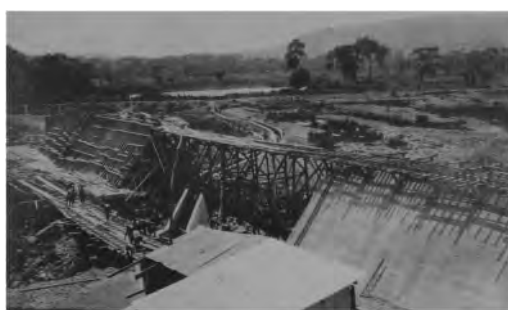
Figure 4. Concreting the gravity dam at Mwadingusha in 1928 (Note documentaire 2 1929).
