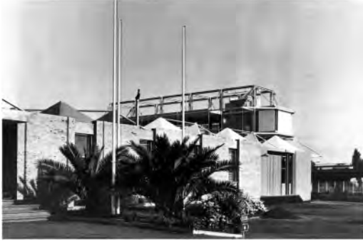
Figure 3. The Angus factory in Casavatore, Naples, M. Pica Ciamarra, 1961–1967 (Courtesy of Pica Ciamarra Associati).
