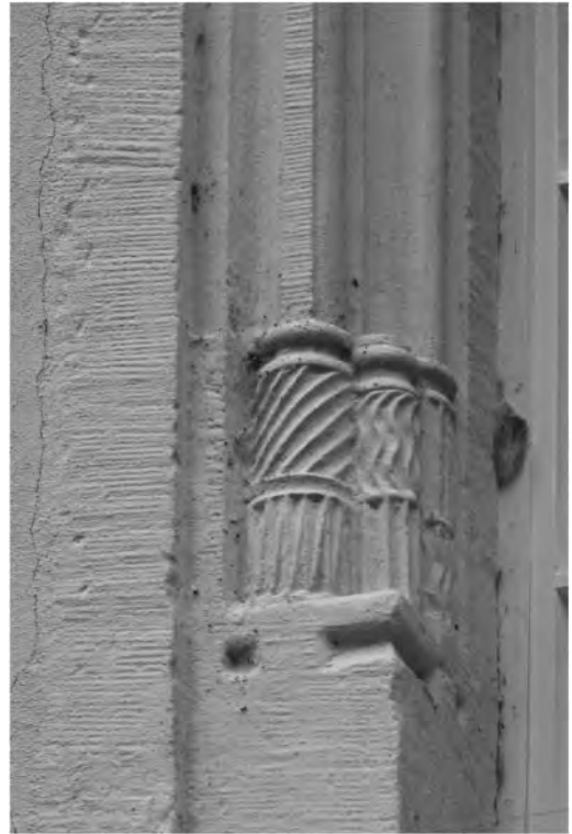
Figure 7. The window jamb in Friedhofgasse No. 11 shows Gothic features and processing traces of a wide chisel. (author 2020).
