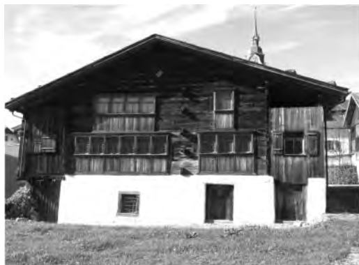
Figure 5. So-called “Haus Bethlehem” Schwyz, Canton of Schwyz. The building logs of this House are dated to 1287 by dendrochronology. Note that the windows as well as the arbors are not original to the medieval building (Gantner 2013).
