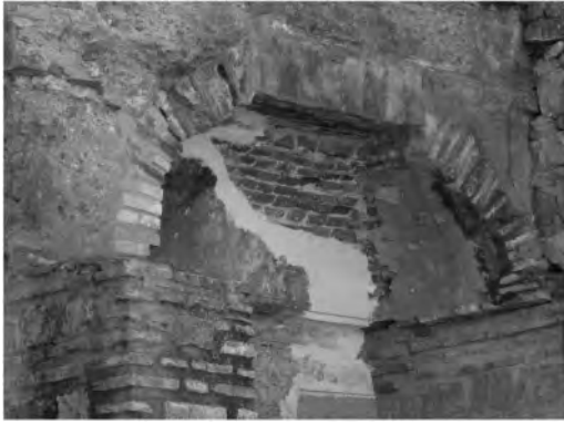
Figure 5. Brick vault in the palace of the Sultan of Tlemcen, Algeria (photograph by Ignacio Javier Gil Crespo).
