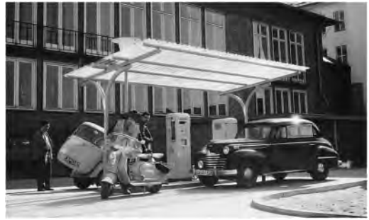
Figure 6. Extruded corrugated transparent Plexiglas roof of a gas station at the Technische Hochschule, Darmstadt 1957 (Photo: Evonik Industries AG, Corporate Archives, Record Group Röhm, Photo Archives, Hanau).
