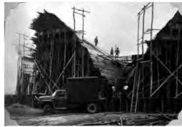
Figure 22. Under construction and recently removed formwork (photos by Laercio Almeida 1980).
