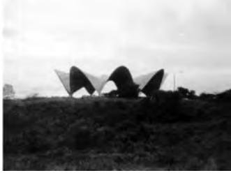
Figure 23. Under construction and recently removed formwork (photos by Laercio Almeida 1980).
