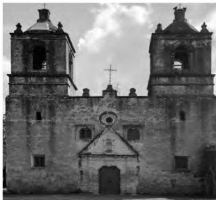
Figure 3. Concepción façade (photo by the authors).
