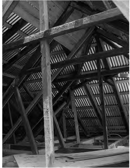
Figure 7. Structure of the hip roof of the Riefkohl-Manautou house in Arroyo (photo by author).
