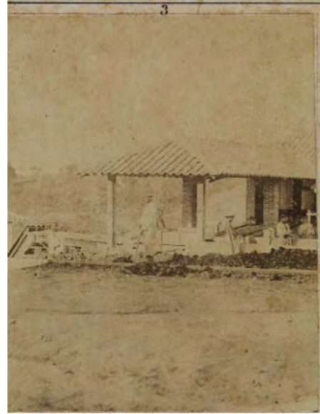
Figure 6. Part of the brick factory from where the bricks were transported to the furnace. Date: 1869. Collection from the Brazilian National Library. Available at: http://acervo.bn.digital.bn.br/sophia/index.asp?codigo_sophia=42170 . Accessed 26 November 2020.
