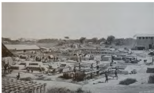
Figure 2. The prefabrication workshops in Lubumbashi, ca 1928 (Trabeka ca 1930).
