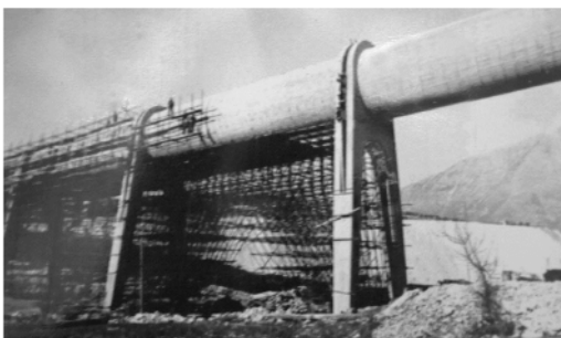
Figure 10. The scaffolding over the Casilina road (ASE).
