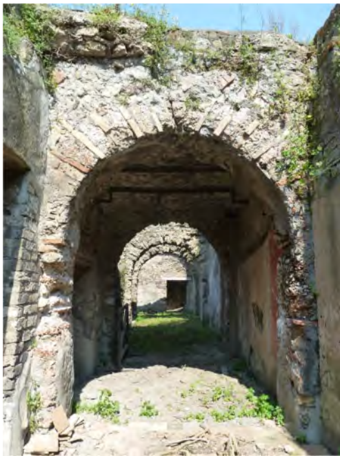
Figure 3. View from the east of gallery N°. 45 with its concrete floor; in the foreground with the arch buttress built in 1774 (Hélène Dessales 2011).
