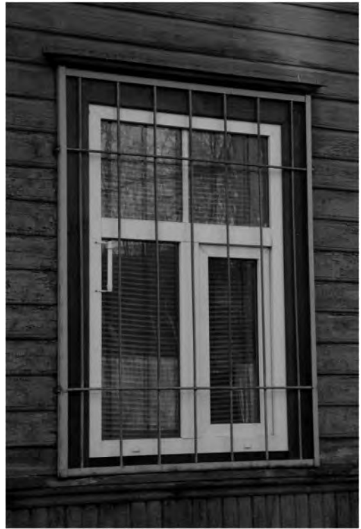
Figure 7. Plastic windows were desirable in 1990s and many original wooden windows were replaced by them.
