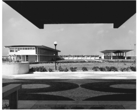
Figure 2. The Montecatini plant in Brindisi, E. Sgrelli, 1960–64 (Courtesy of Archive Giordani, Malaguzzi, Valeri e Sgrelli).
