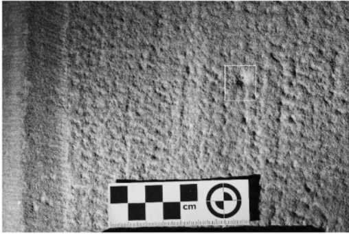
Figure 6. The pillar in the Kornschütte of the town hall in Lucerne show traces of a pointed chisel and a serrated tool. (author 2019).
