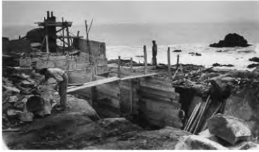
Figure 1. Boa Nova Tea House and Restaurant, concrete foundations, 1959 (Câmara Municipal de Matosinhos).
