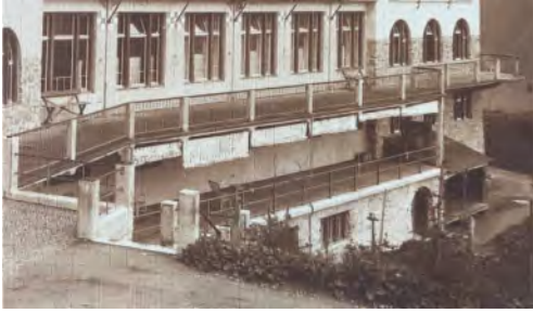
Figure 4. The public cantilevering terrace in the ground floor that evolves into the curved Consolenplatte (source: Staatsarchiv Thurgau StATG 9'11, 10.4/0).
