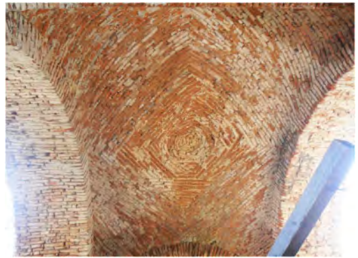
Figure 9. Vault under the bell tower of Comana monastery in Romania (photograph by Ignacio Javier Gil Crespo).
