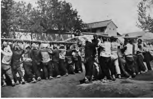
Figure 3. Xinjiang Cathedral, earth-ramming works on the site, 1936 (© Het Utrechts Archief, 1224, 291/48).
