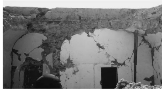
Figure 8. Upper cloister, remains of both vaults. Photo taken in 2017.
