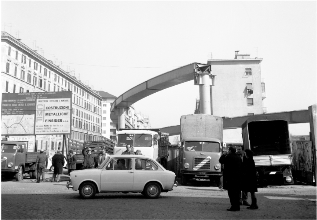
Figure 11. Rome flying road during the construction, 1969–1972 (Riccardi Historical Archive).
