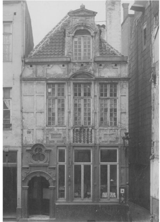
Figure 6. The facade of the Gouden Huyve situated in Rue de l'Etuve 13 was carefully dismantled in the 1920s and reconstructed in 1929 next to Sint-Nicolas Church. Collection Comité d'Etudes du Vieux Bruxelles . © KIK-IRPA Brussels.
