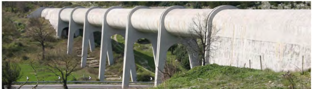
Figure 13. View of the bridge in 2014 (source: the authors).
