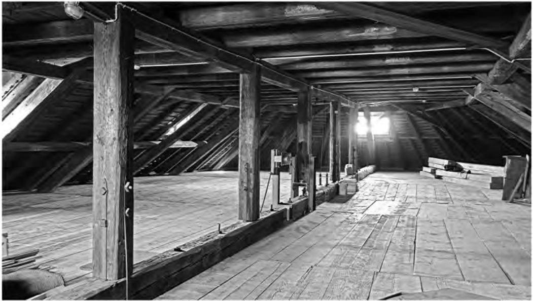
Figure 3. Roof construction of the church (Schäfer 2019).
