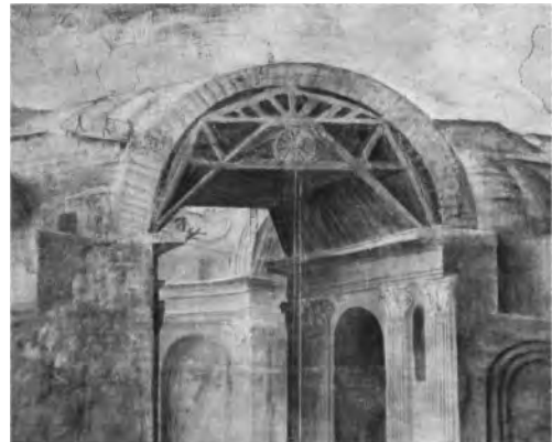
Figure 1. Vasari's fresco (detail) of 1546 in the Sala dei Cento Giorni , Cancelleria, Rome, showing the erection of the brick barrel vault on the southern arm of St. Peter's Basilica, Rome (author).
