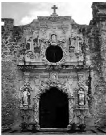
Figure 5. San José façade (Photo by the authors).
