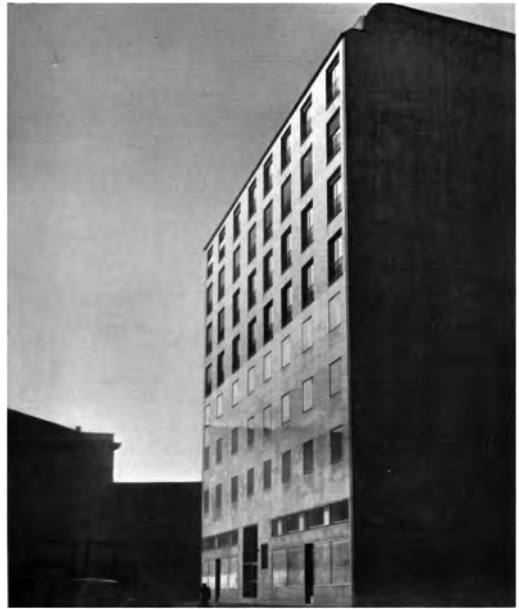
Figure 3. Building in via Velasca by Asnago & Vender, 1950. Source: Bottoni 1954.
