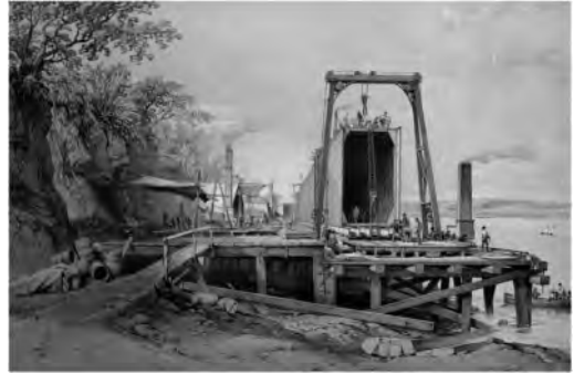
Figure 2. Construction of the Britannia Bridge (Clark 1850).
