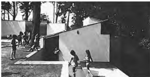
Figure 4. Quinta da Conceição swimming pool, changing rooms 1965 (Trigueiros 1997, 43).
