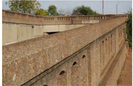
Figures 4(top) and 5(bottom). MacArthur Bridge guardrail and Chippewa street underpass.
