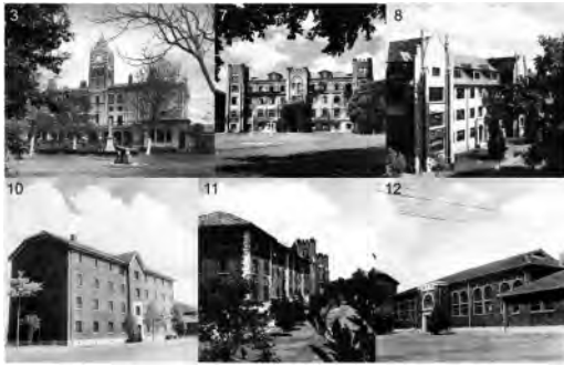
Figure 6. Buildings of the quadrangle, Soochow campus (source: Special Collections, Divinity Library, Yale University, United Board for Christian Higher Education in Asia, RG011-415-5874-5014; 5002; 5003; 4999; 4998; 5001).
