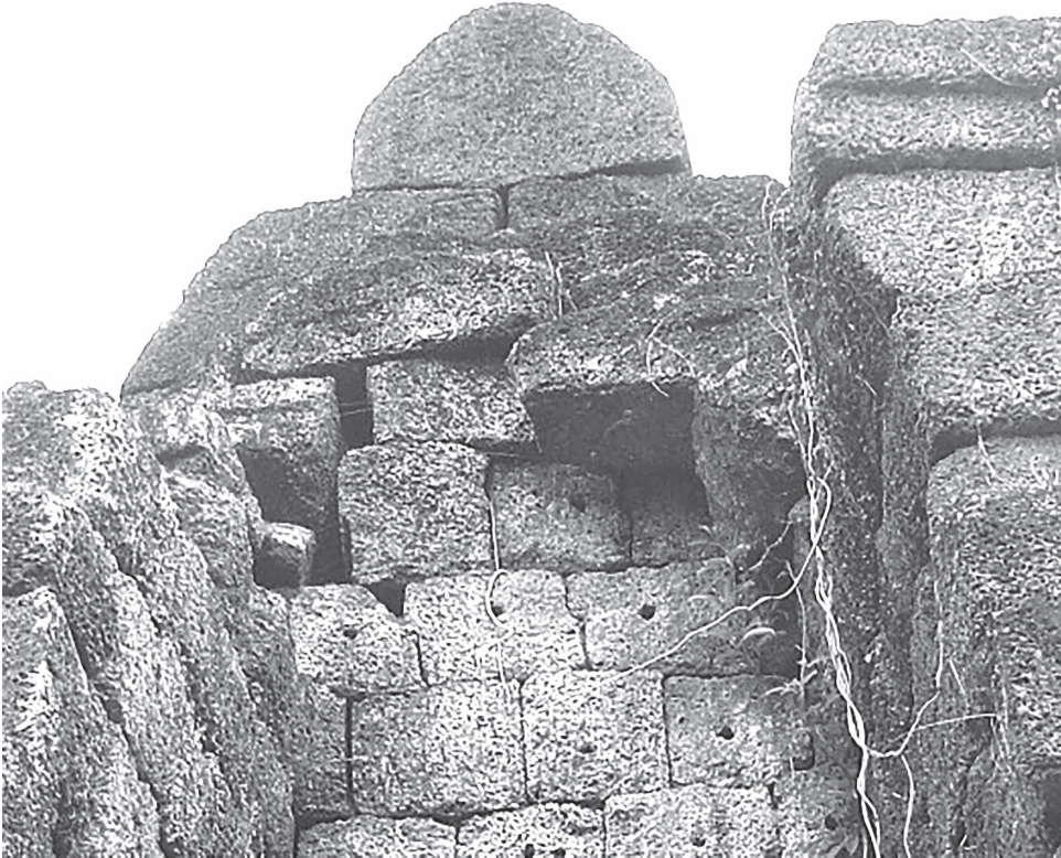
Figure 2.6 Detail of vertical ‘bayonet-cut’ joints in the corbelled vault from prasat tower ρ in Preah Khan of Kompong Svay.
