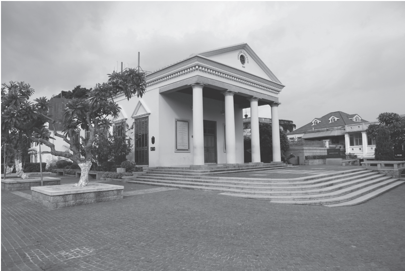
Fig. 6 The Union Church before repairs. Courtesy of Chen Yongpeng.
