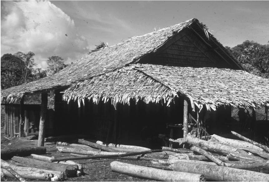
Figure 8.2 Large cocoa fermentaries, such as this one at Hukuha (1975), used enormous amounts of high quality timber.
