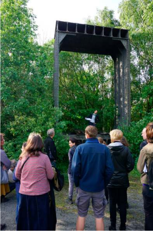
Remains of the old Britannia Bridge Structure, staging Balke calling colleagues to increase productivity (Bangor, 2019). Reproduced with permission © Huw Jones
